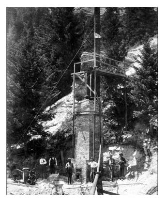
The first oil shale retort in Colorado, shown here in a photograph printed in National Geographic in 1918, was built by the Oil Shale Mining Company on Dry Fork west of De Beque, Garfield Country, Colorado. Designed from illustrations found in the *Encyclopedia Britannica* entry on the Scottish oil shale industry, the retort heated crushed shale to extract oil. Credit: US Geological Survey
