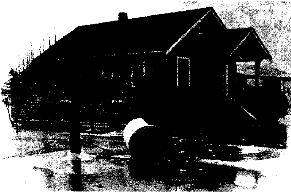
Figure 7. Propane Tank Deposited Next to Home by Flood.
