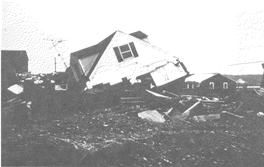
Severe damage in Scituate, Massachusetts, caused by the February 1978 "Northeaster."
