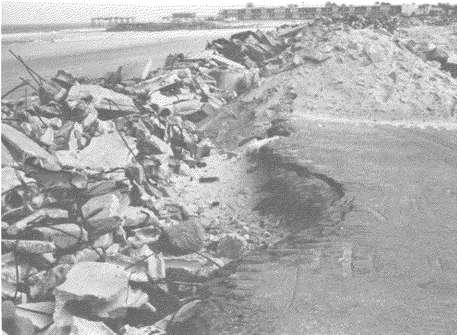
Flood and erosion-damaged road, St. Augustine, Florida.
