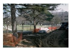
Figure 6: Construction vehicles can damage the existing soil structure by compressing soil particles.
