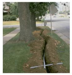
Figure 5: Trenching near trees can severely damage root systems.
