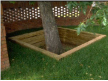
Figure 2: Tree wells cannot compensate for the addition of soil over tree roots.
