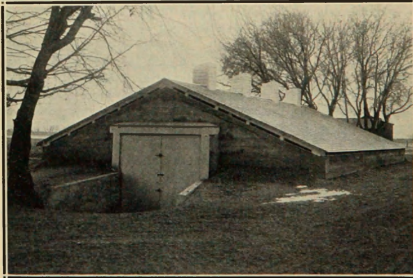
Fig. 4—Potato storage house at experiment station.
