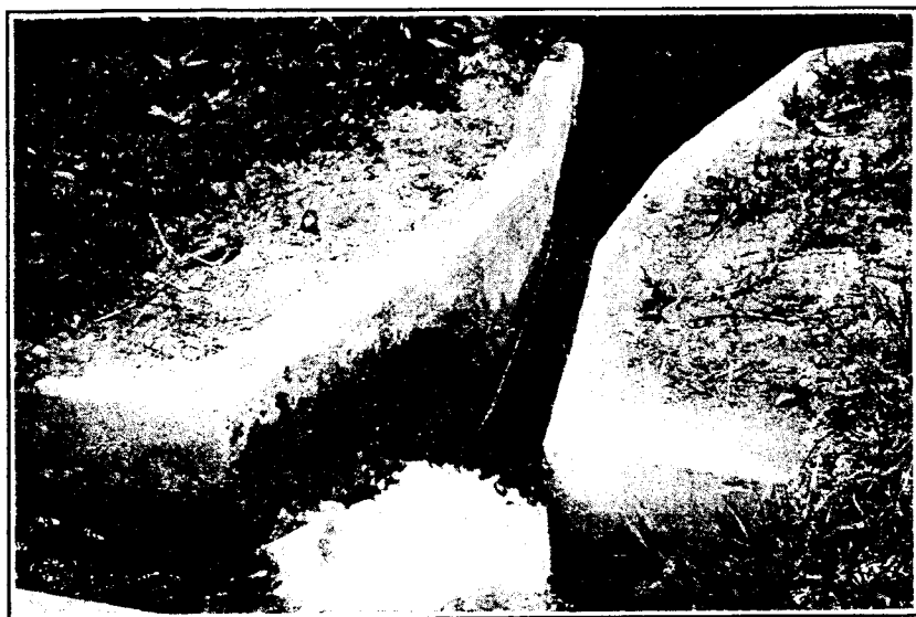
Figure 23.—One-foot reinforced concrete Parshall measuring flume, free-flow discharge of 4 second-feet. Lake Canal, near Fort Collins, Colo.
