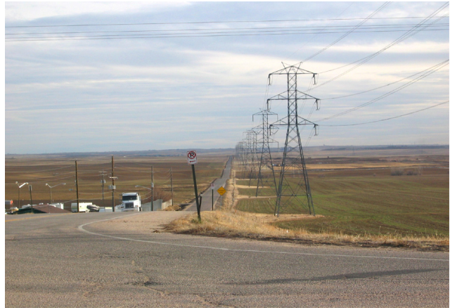
View south of the Powhatan Road overpass. Power lines and agricultural land uses dominate the middleground and background views.
