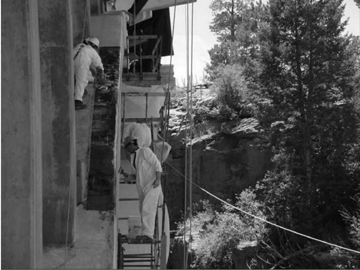
Figure 1-6 Applying Fibrwrap to arch Extrados
