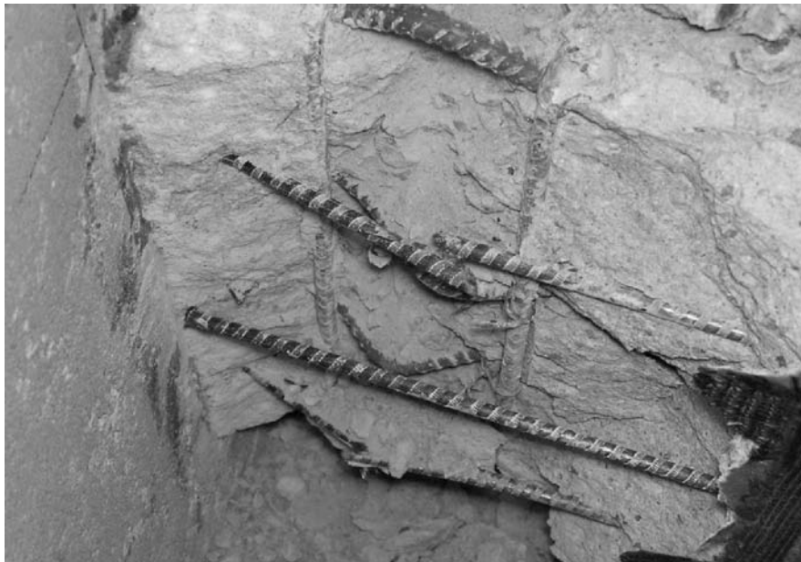
Figure 1-67 Buckled rebars and ruptured Leadline at the top of the FR critical section (Note: specimen is lying on its side and loose debris has been cleared away.)
