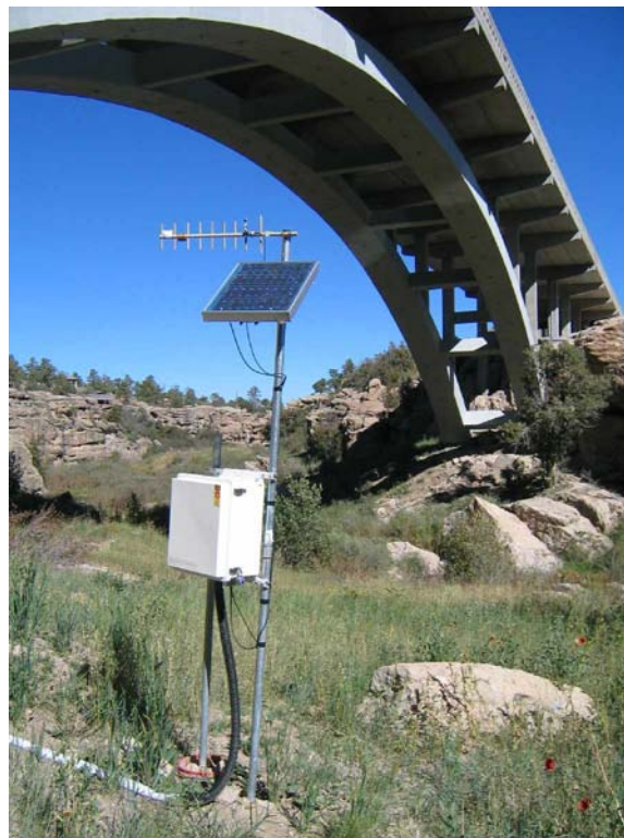
Figure 3-4 In-situ health monitoring system in Castlewood Canyon Bridge
