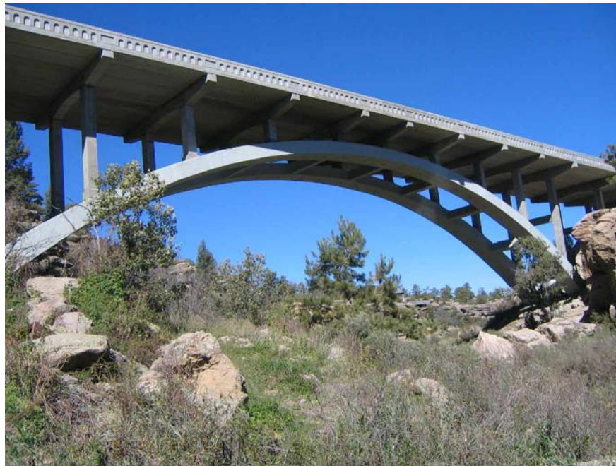
Figure 3-1 The repaired Castlewood Canyon Bridge
