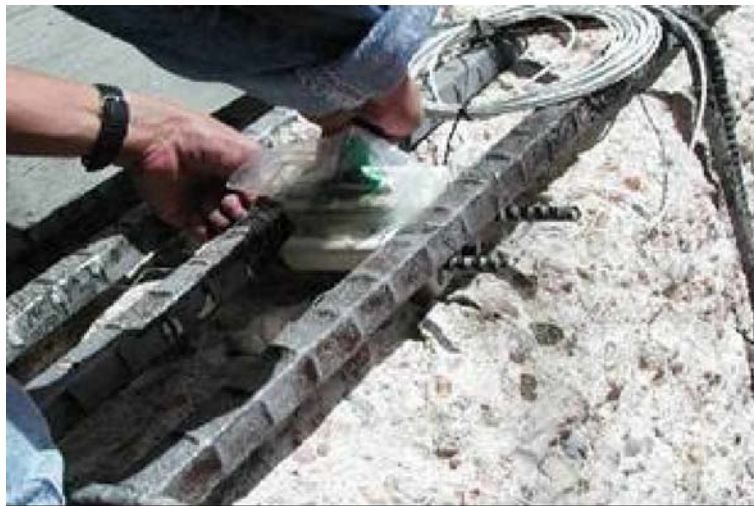
Figure 3-9 Installation of corrosion sensors during construction
