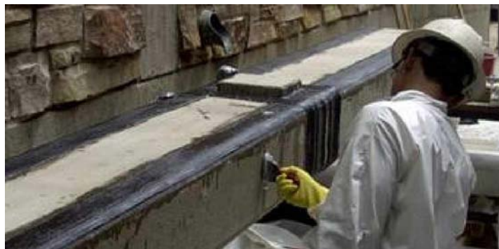
Figure 2-8 Epoxy overcoating in progress
