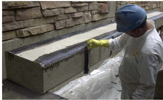
Figure 2-7 Placing CFRP sheet on concrete in progress
