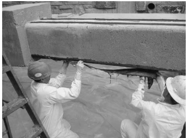
Step 4: Applying Fibrwrap
