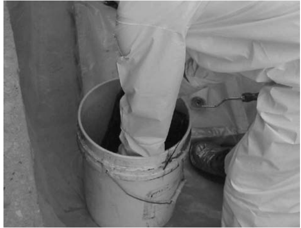
Step 2: Saturating Fibrwrap in epoxy
