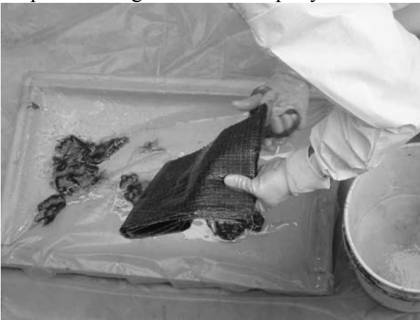
Step 3: Trimming saturated piece
