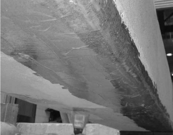
Step 1: Wetting surface with epoxy
