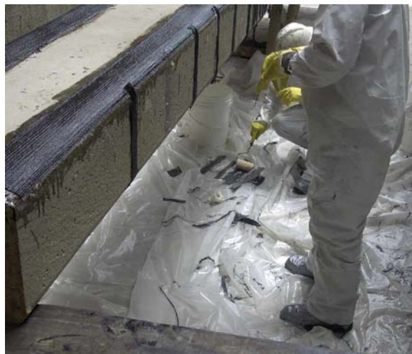
Figure 2-6 Epoxy undercoating in progress
