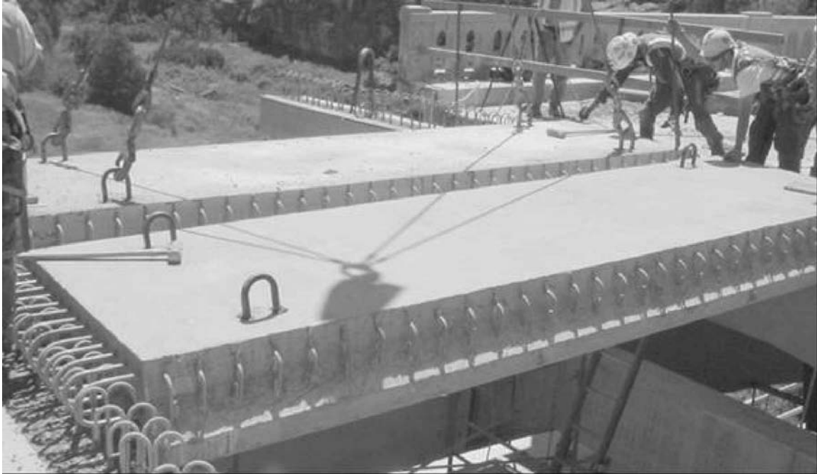
Figure 1-8 Precast deck panels
