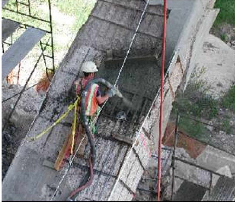
Figure 3-12 Shotcreting over corrosion instrument
