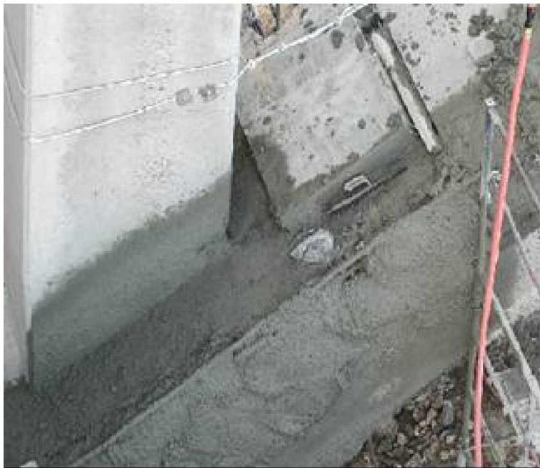
Figure 3-13 The embedded corrosion instrument (ECI-1)
