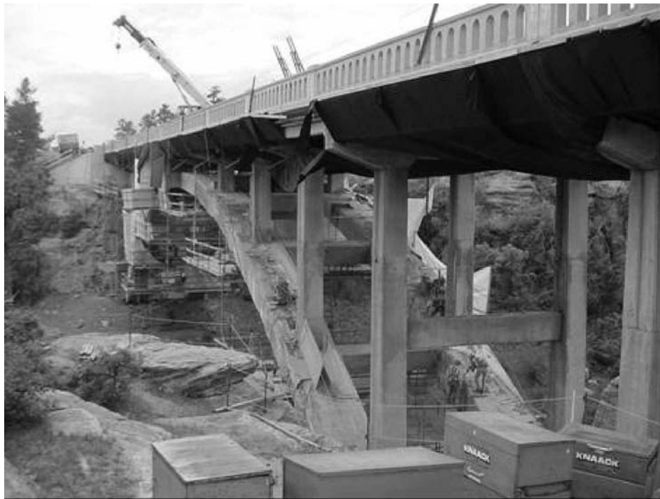
Figure 1-5 Arches during construction
