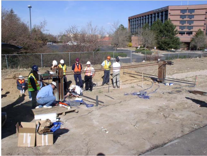
Figure 5.47 Picture showing the installation of the testing devices
