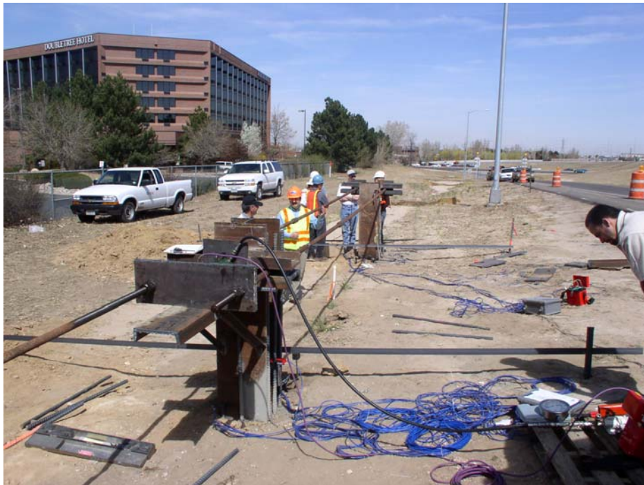
Figure 5.52 Running the test and watching the instruments
