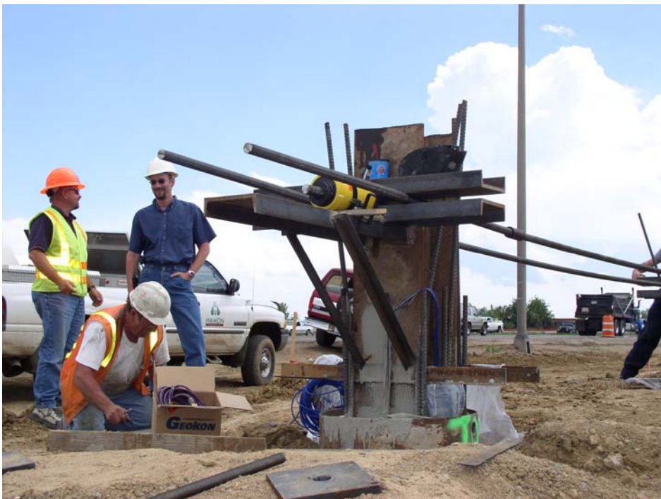
Figure 5.10 Picture showing the installation of the testing devices
