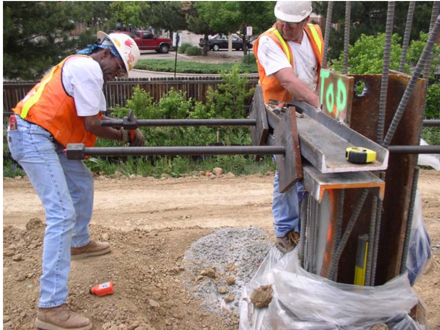
Figure 5.11 Picture showing the installation of the testing devices
