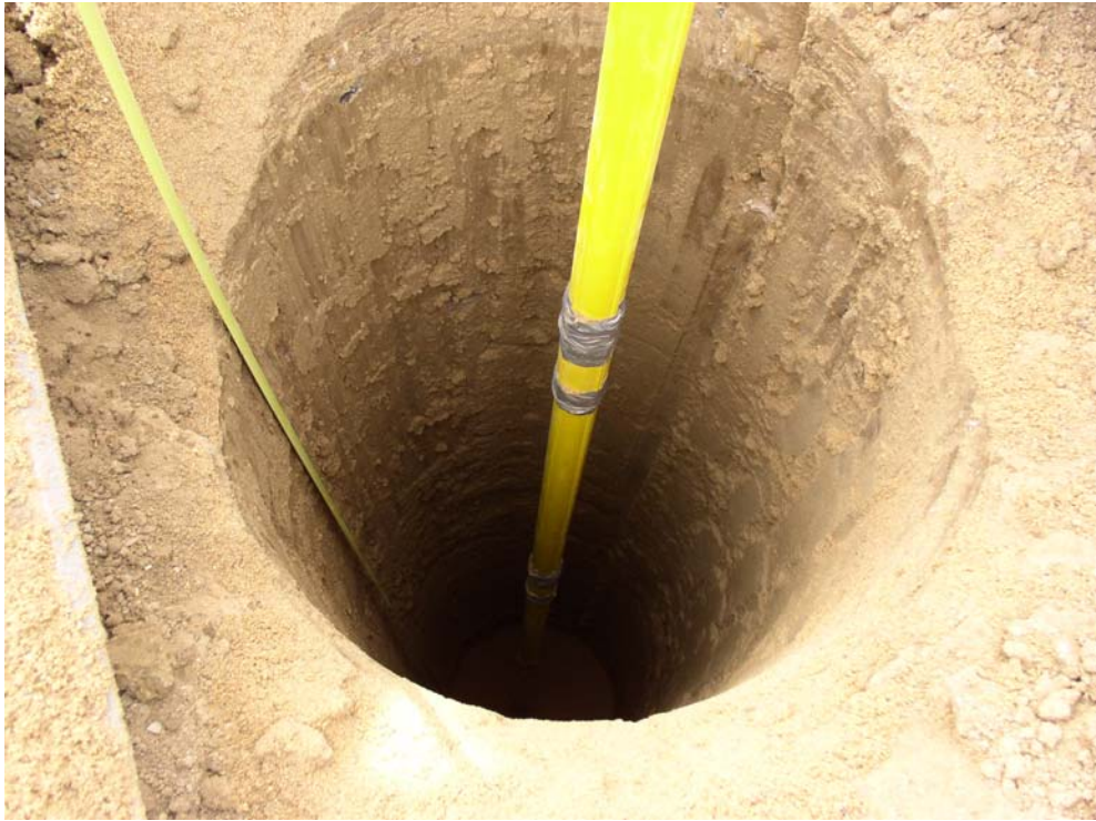
Figure 5.5b Inclinometer installation in the hole
