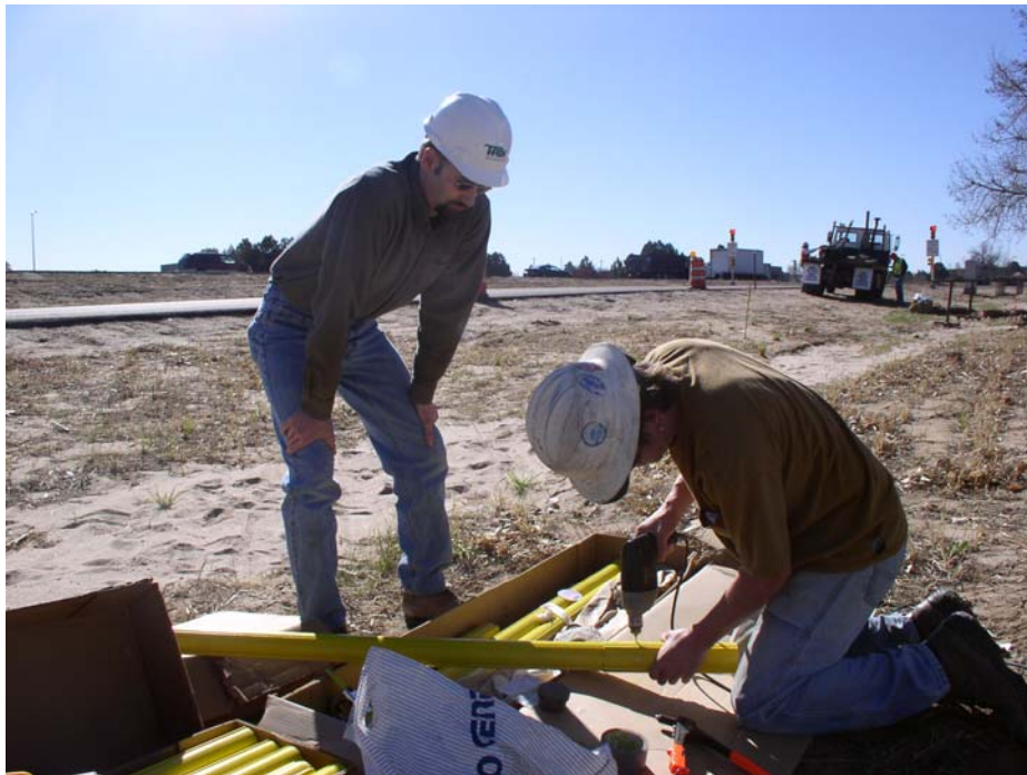
Figure 5.40 Installation of gage on steel cages
