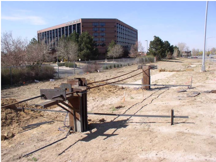
Figure 5.46 Picture showing the installation of the testing devices
