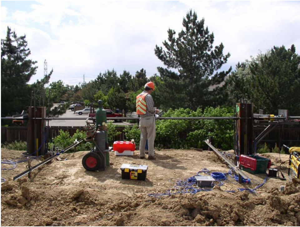
Figure 5.15 General view of the load test
