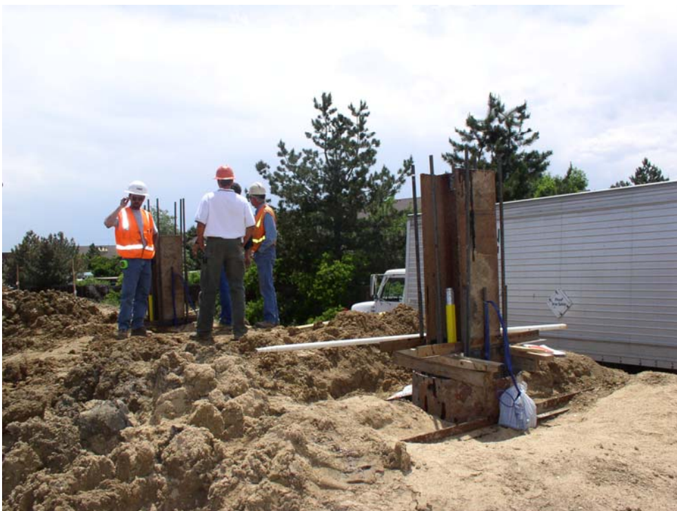
Figure 5.8 Drilled shafts installed and ready for concrete
