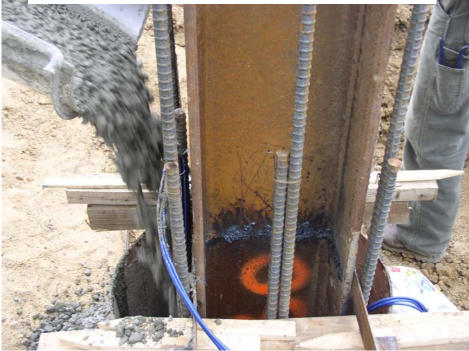
Figure 5.9 Pouring concrete in the hole
