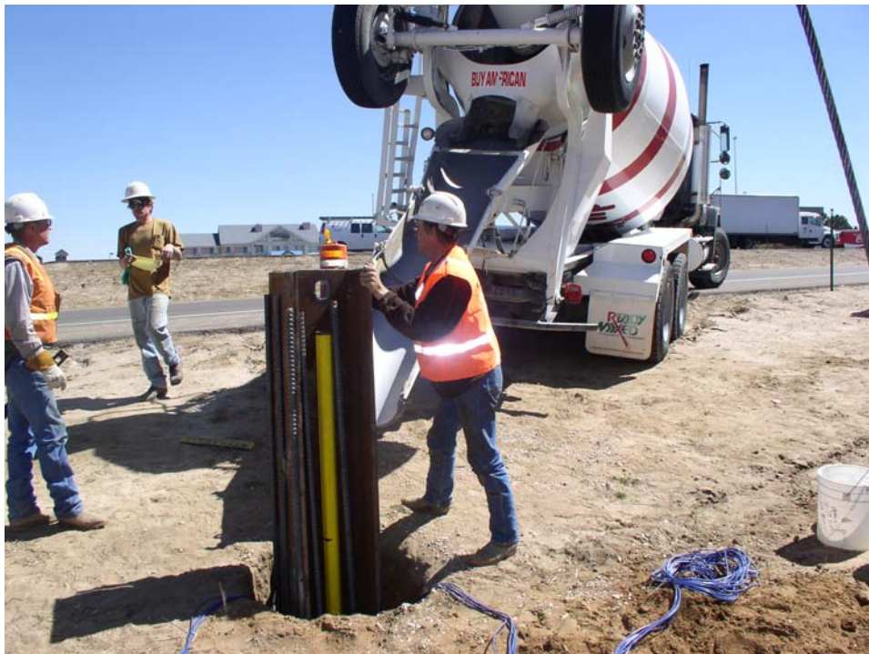
Figure 5.44 Drilled shafts installed and ready for concrete
