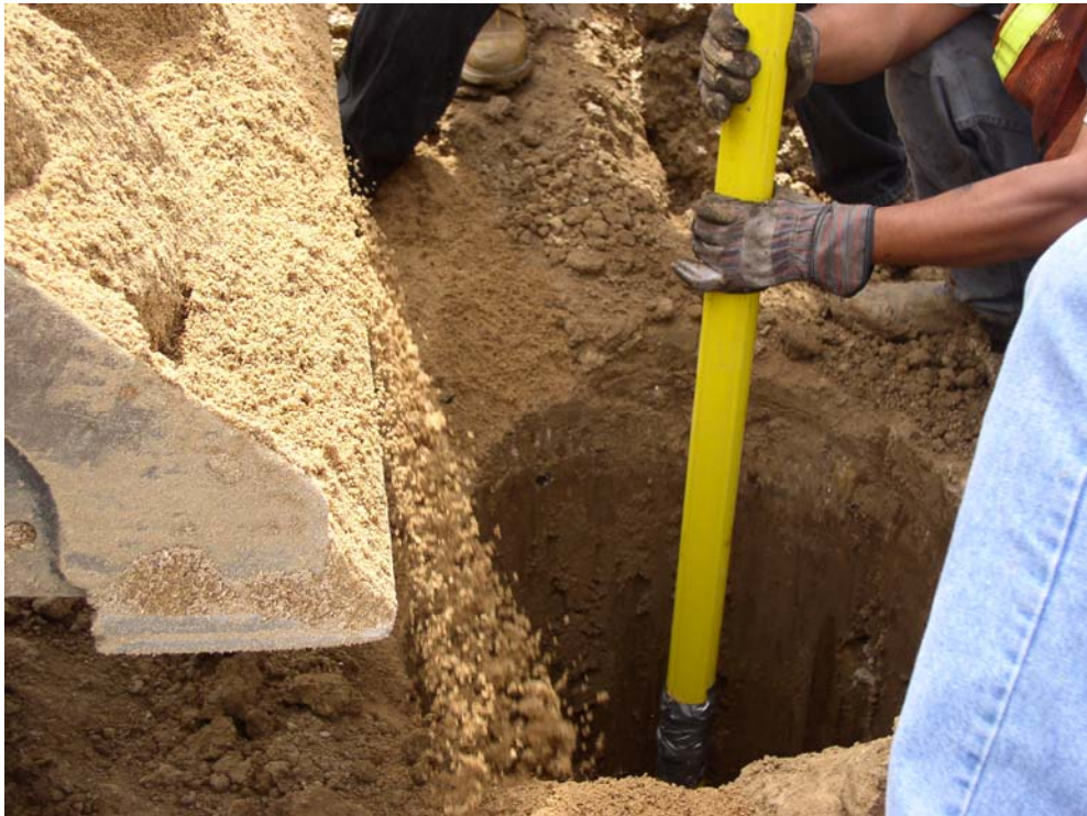
Figure 5.6 Pouring sand to fill around the bottom 6' of the inclinometer tube
