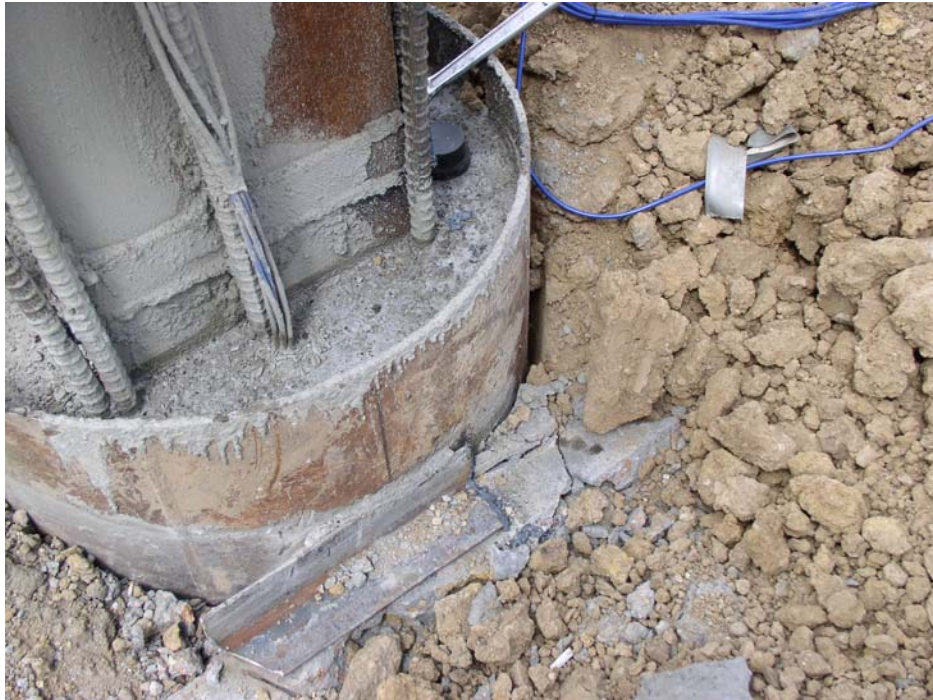
Figure 5.17 Picture showing opening behind the shaft during the test
