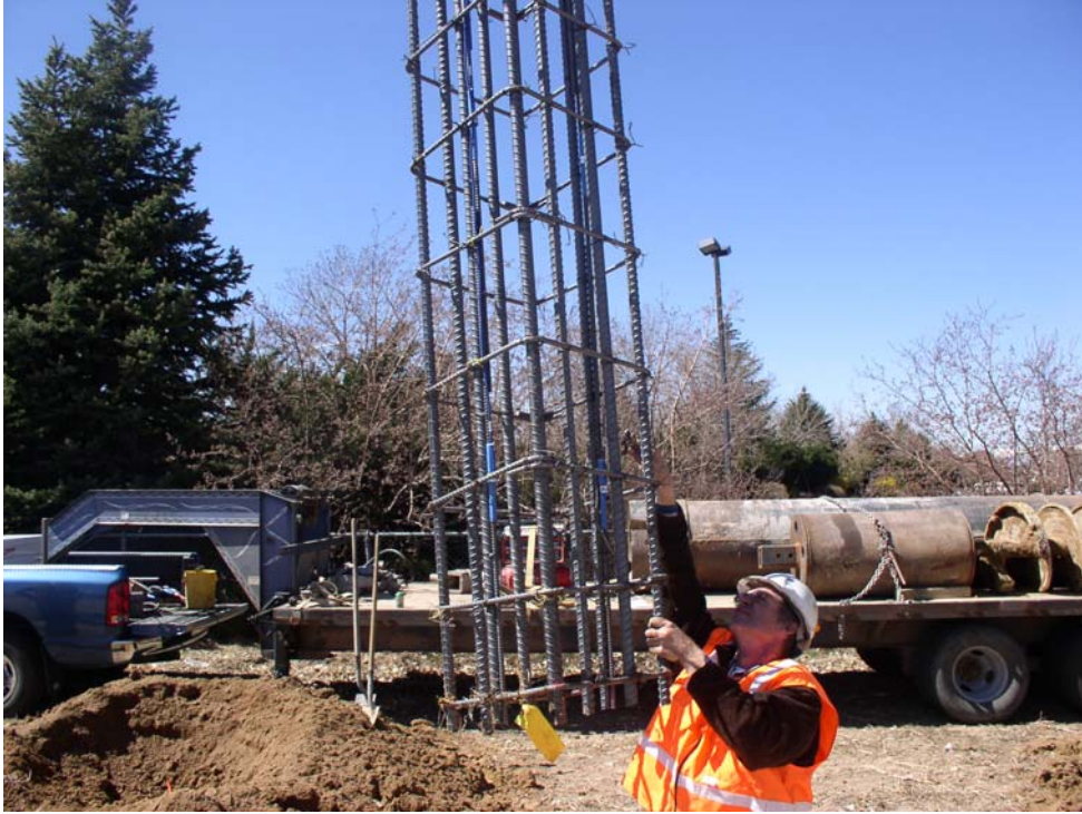
Figure 5.43 Instrumented cage transferred to the hole
