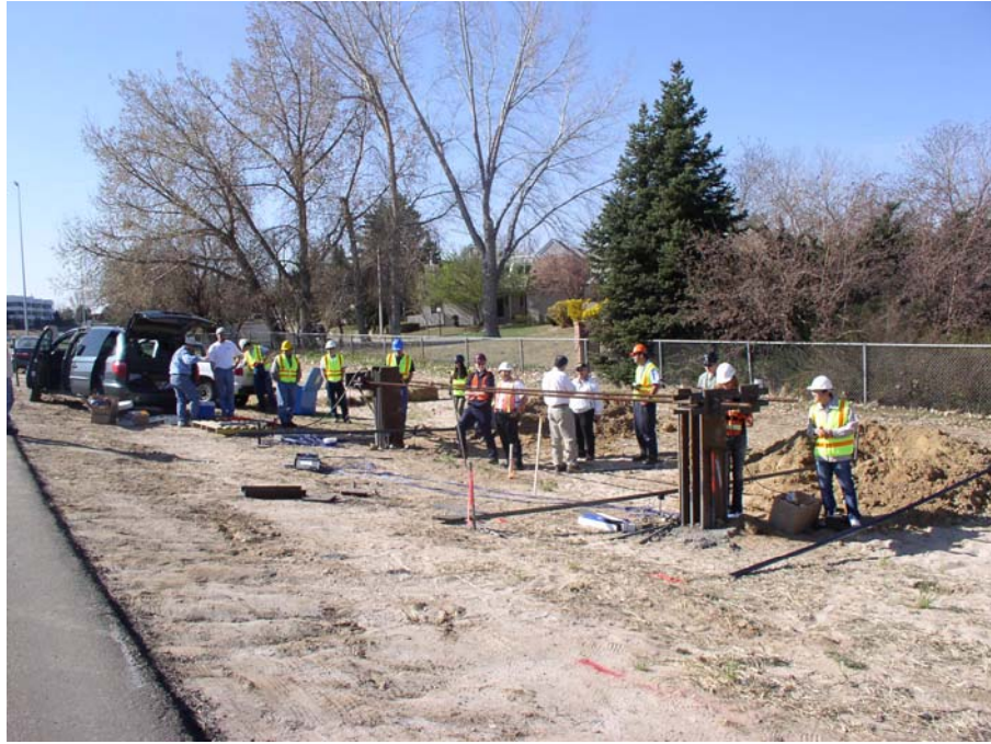
Figure 5.51 General view of the load test
