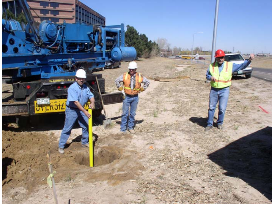
Figure 5.41b Inclinometer installation in the hole
