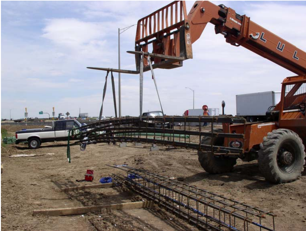
Figure 5.7 Instrumented cage transferred to the hole
