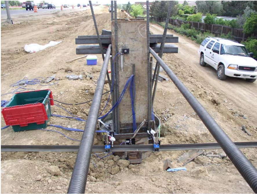
Figure 5.13 Setup of measuring devices at shaft 2 (South)
