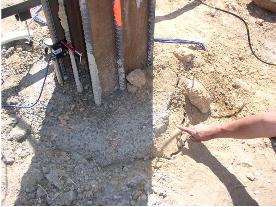
Figure 5.53 Picture showing opening behind the shaft during the test
