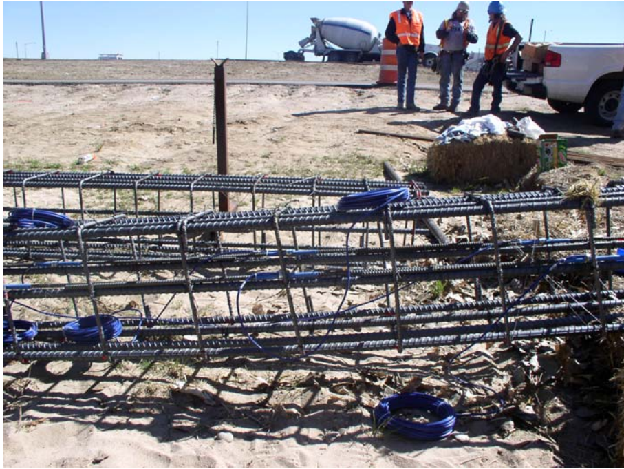
Figure 5.40 Installation of gage on steel cages
