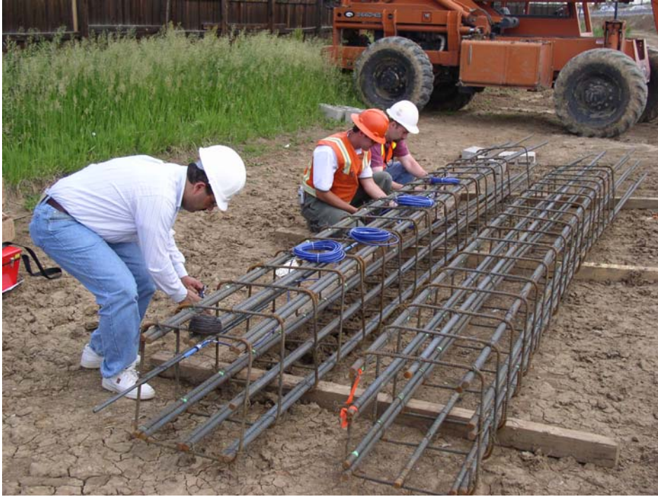
Figure 5.4 Installation of gage on steel cages
