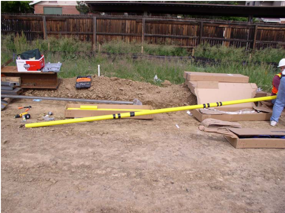
Figure 5.5a Inclinometer assembly
