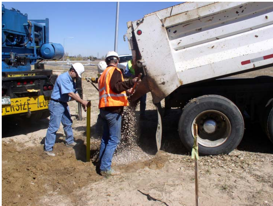
Figure 5.42 Pouring sand to fill around the bottom 6' of the inclinometer tube
