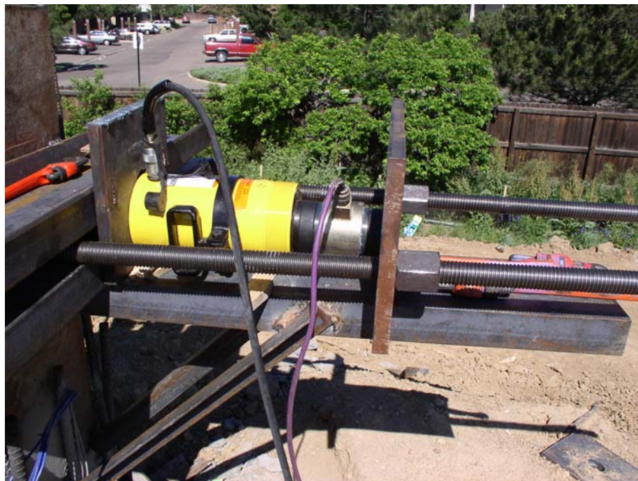
Figure 5.12 Picture showing the jacking devices
