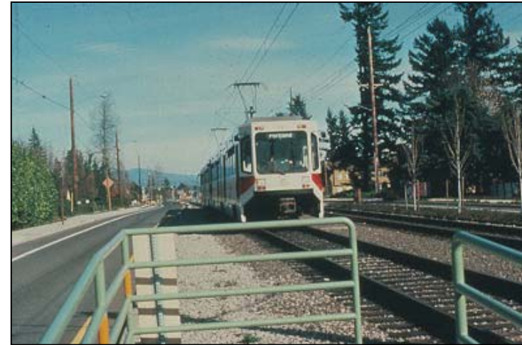
Figure 3w. A Portion of the Portland Light Rail System Runs on Freight Tracks, a Preserved Right-of-Way
