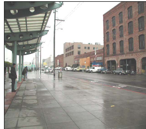
Figure B3. Renovation of Industrial Buildings to Residential Units at San Francisco Station
