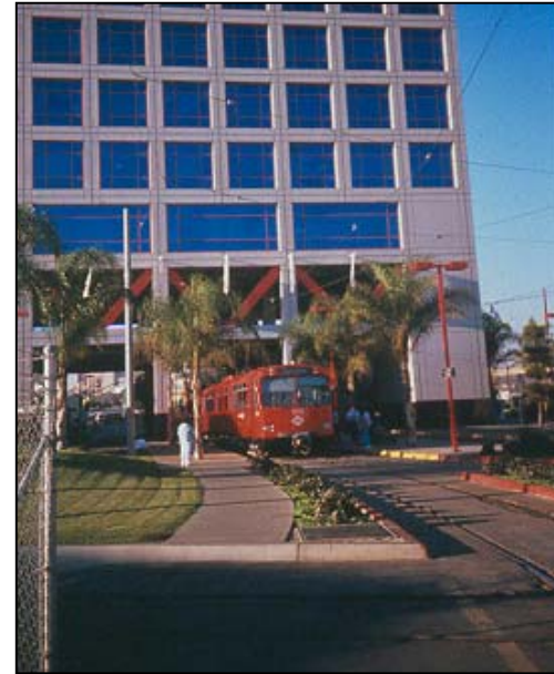
Figure 3v. One of the Stations of San Diego’s Light Rail System was Incorporated into a Building, which Involved a Creative Approach to Maintaining the Public Right-of-Way
