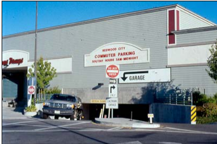
Figure 3j. Parking Facility at Station Area
