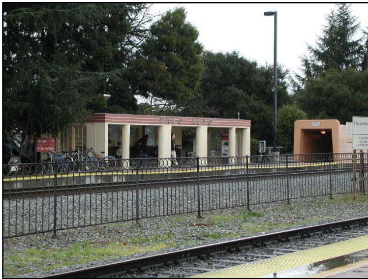
Figure 3s. Bus Stop Located Outside of Palo Alto Caltrain Station
