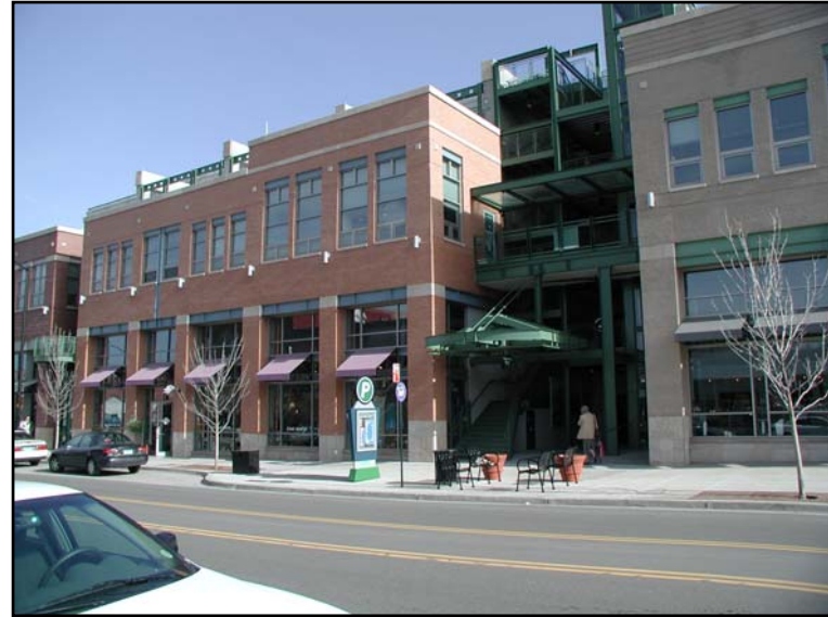
Figure 3t. Example of a Structured Parking Facility that Fits in with its Adjacent Downtown Environment
