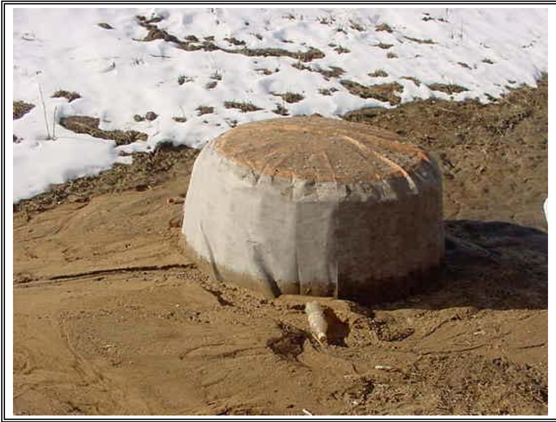
FIGURE SC 4.5 Rigid Inlet Protection Device
