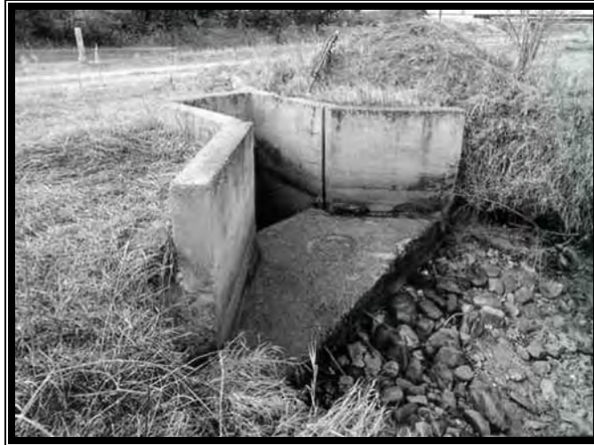
Cottonwood Ditch #2 north side of Arapahoe Road
