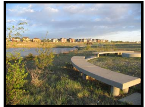
Picnic benches and other public open space amenities are commonly located in stormwater detention facilities.
