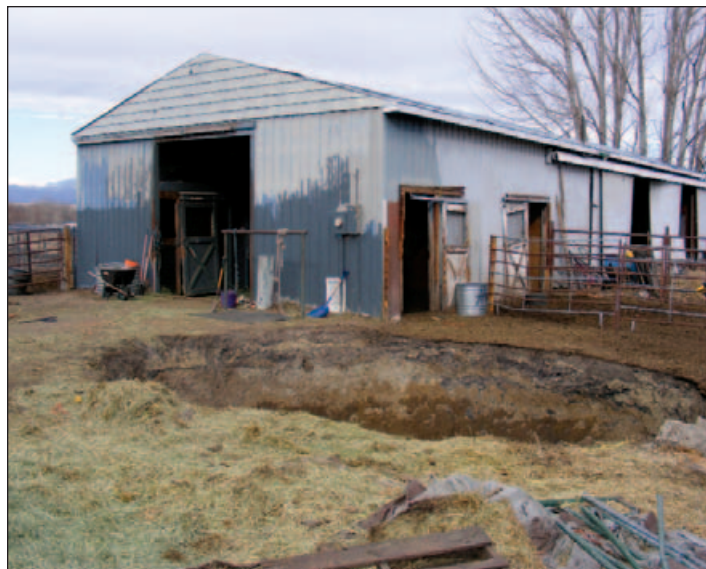
A sinkhole caused by subsidence of an old coal mine east of Erie in 2009. The MSIC maintains a database to assist landowners and developers identify areas where subsidence could present a problem.
