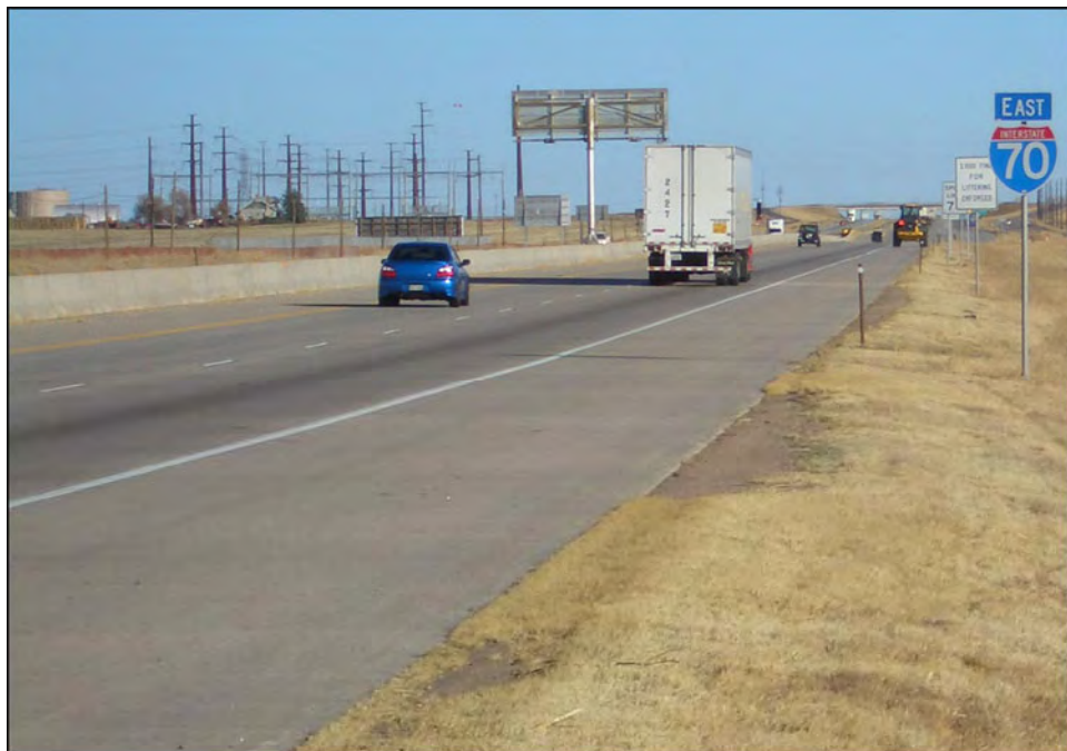
Figure 3-2. The I-70/E-470 testing site
