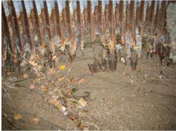
Figure 7. Culvert pipe corrosion near Castle Rock, I-25
