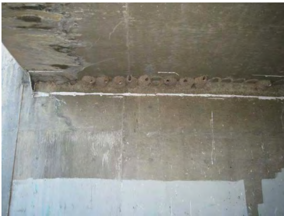
Figure 3. Nests in Northernmost CBC where Corner Slopes Have Blown Down.
