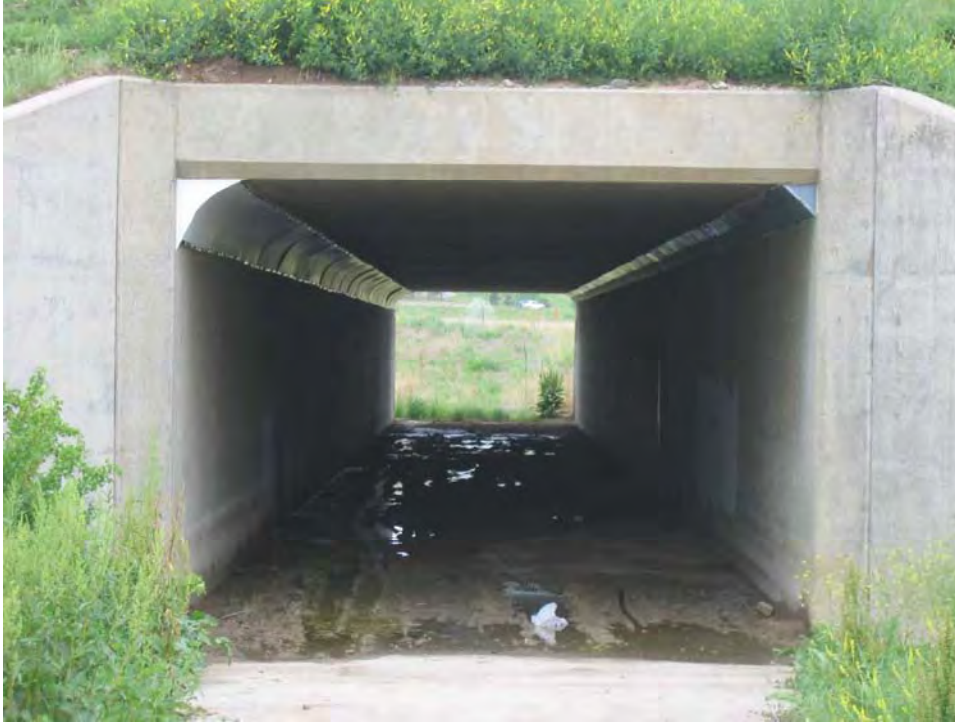
Figure 14. Looking west in CBC 4 with corner slope deterrents in place.
