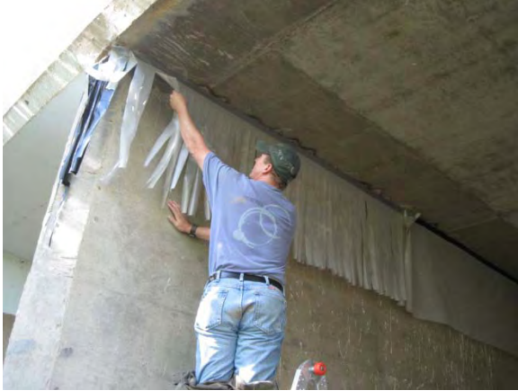
Figure 7. Jeff Peterson Removing Plastic Strips from Lath.
