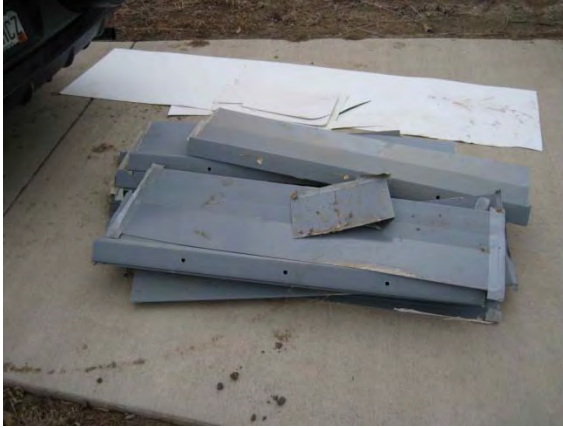
Figure 17. Bird Slide panels and white plastic panels collected after December 2008 wind storm.
