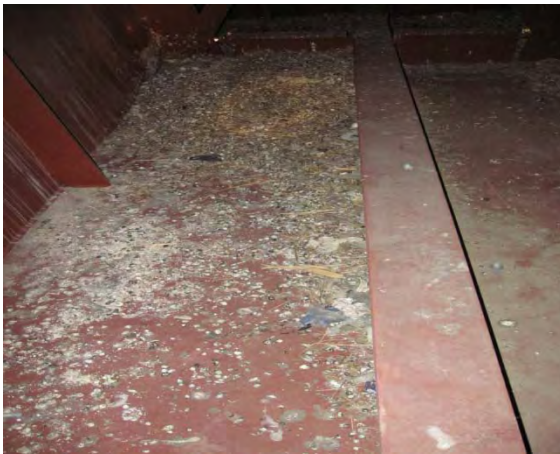
Figure 4. Pigeon feces in Gir 5A where pigeons entered through 3-inch gap.
