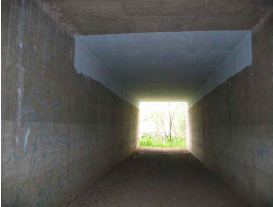
Figure 11. Looking east from within CBC 1 (southernmost) with blue ceiling.
