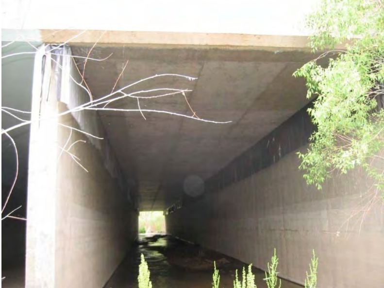
Figure 12. Looking west in CBC 2 with plastic strips installed.
