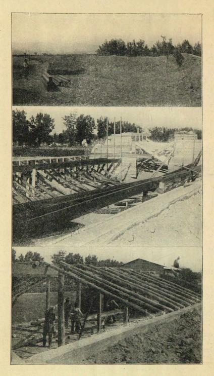
PLATE XVI.-The Station Cellar. Excavation. Braced Concrete Forms. Framing the Roof.
