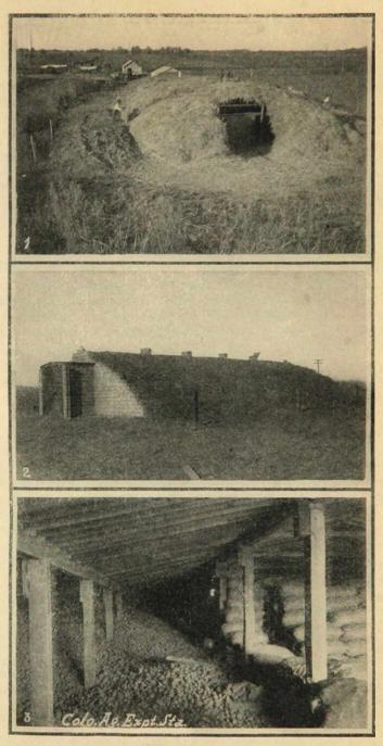
PLATE XVII.—Potato Cellars 1. Strawing. 2. Exterior. 3. Interior.
