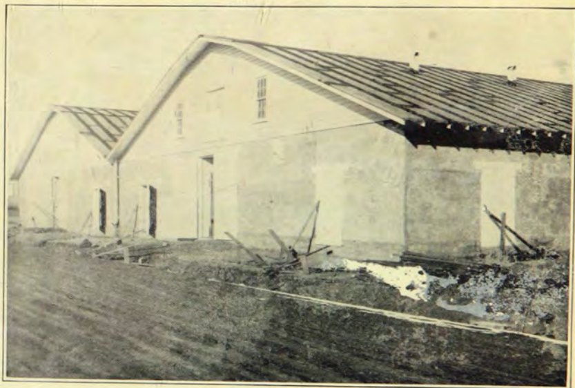
Fig. 9.—A double-walled adobe storage house with air space between walls and ventilators in roof. This house was successfully used for onion storage.
