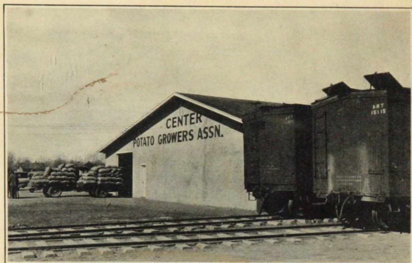
Fig. 68. Trackside storage and grading plant.
