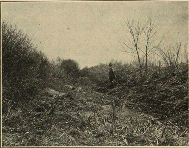
Fig. 3—An irrigation ditch heavily overgrown with tall weeds.
