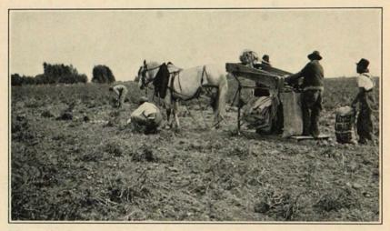
Figure 80. Sorting potatoes in the field. The picker should hold the basket close to the screen, and the sorter should not be shaken while the picker is dumping.
