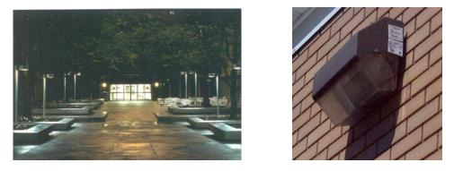
Figure 4. Fully shielded or IESNA full cutoff luminaires (left) are recommended. Do not use unshielded floodlights or wallpacks (right).
