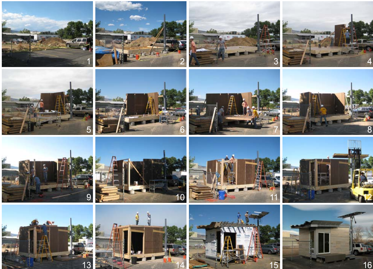
Time lapse showing the BioSIP installation process
