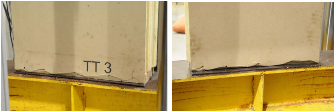
Photo 1.5: Detail showing failure of BioSIP Axial #2 test prototypes at: (left) interior face of panel skin at sill plate connection, and (right) at exterior face of panel skin at sill plate connection.
