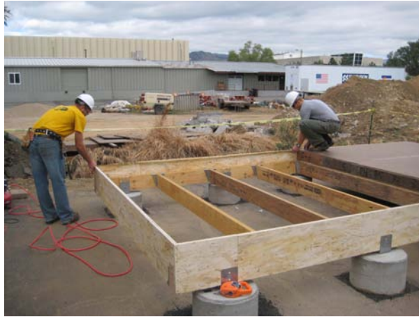
Prefabricated solar tracker column being set onto concrete foundation (above left). Final dimensions were verified before BioSIP floor panels were set in place (above middle). Kellen Schauer mann checking precision of BioSIP wall panel during installation (above right).
