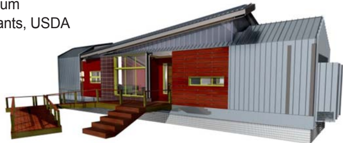
CU's 2005 Solar Decathlon home was constructed with first-generation BioSIPs, a standard sandwich panel SIP invention.
