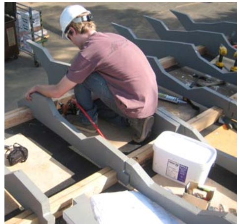
BioSIP Research Structure with BioSIP floor, wall, and roof panel enclosure in place and ready for installation of exterior finishes (above left). CU Bachelor of Environmental Design (B.ENVD) student, Patrick Westfeldt, installing prefabricated roof trusses on BioSIP roof panel enclosure (above center). Roof trusses were fabricated by the CU BioSIP team using diverted waste sources and digital fabrication methods.
