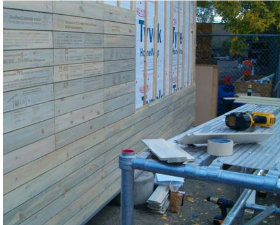
Patrick Westfeldt and Eric Doner standing beneath solar tracker and PV array (above left). Installation of beetle kill siding on building's west elevation (above middle). Kellen Schauermann and Julee Herdt discussing color and finish options with Ryan Chivers (Artesano, LLC) for the eco-mortar finish used around the entry area (above right).
