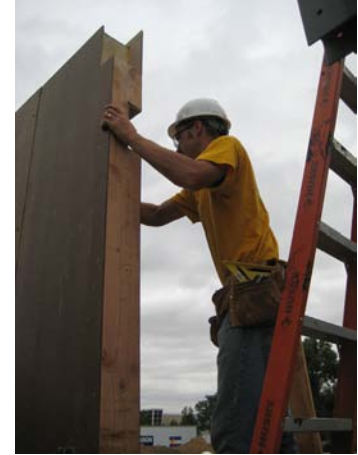
Prefabricated solar tracker column being set onto concrete foundation (above left). Final dimensions were verified before BioSIP floor panels were set in place (above middle). Kellen Schauer mann checking precision of BioSIP wall panel during installation (above right).
