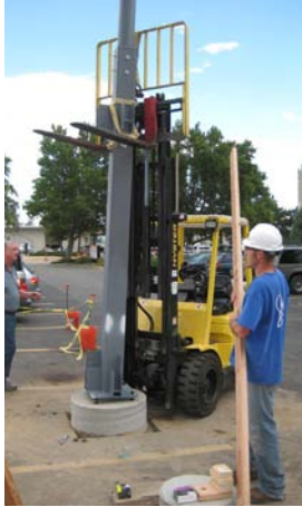
Prefabricated solar tracker column being set onto concrete foundation (above left). Final dimensions were verified before BioSIP floor panels were set in place (above middle). Kellen Schauer mann checking precision of BioSIP wall panel during installation (above right).
