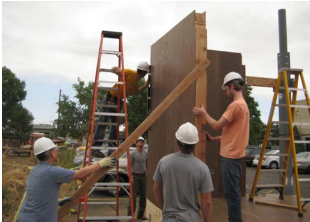
Construction team installing BioSIP wall panels (above left). Special thanks to Michael Honaker, Keaton Schauer mann, Mathew Doner, and Drew Doner for their volunteer efforts during the two-day BioSIP wall, floor, and roof installation.
