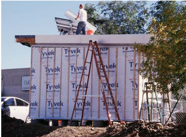
Research Structure with weather barrier installed; metal roof installation in progress (above left). CU Bachelor of Environmental Design students Cullen Taub and Patrick Westfeldt working with Eric Doner to install metal roof finish (above right).
