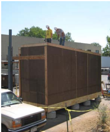
BioSIP Research Structure with BioSIP floor, wall, and roof panel enclosure in place and ready for installation of exterior finishes (above left). CU Bachelor of Environmental Design (B.ENVD) student, Patrick Westfeldt, installing prefabricated roof trusses on BioSIP roof panel enclosure (above center). Roof trusses were fabricated by the CU BioSIP team using diverted waste sources and digital fabrication methods.
