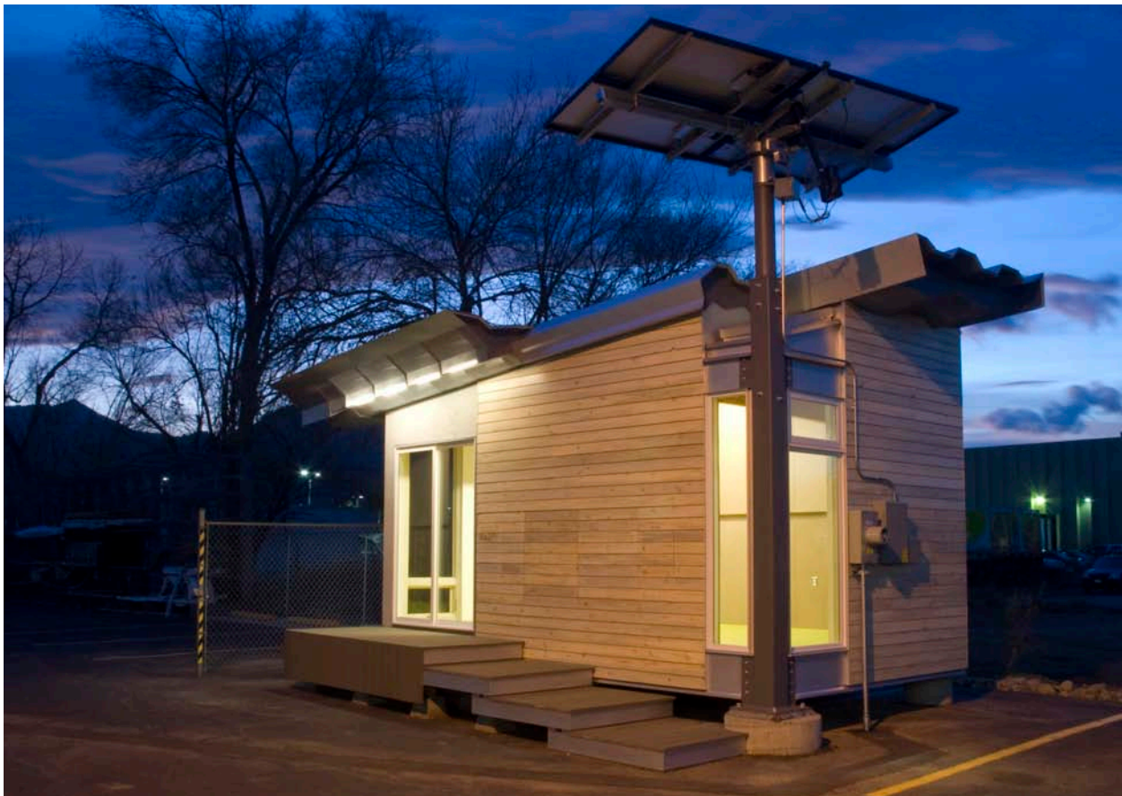
Constructed BioSIP Research Structure
