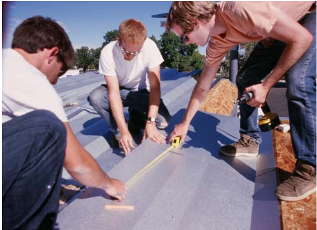
Research Structure with weather barrier installed; metal roof installation in progress (above left). CU Bachelor of Environmental Design students Cullen Taub and Patrick Westfeldt working with Eric Doner to install metal roof finish (above right).
