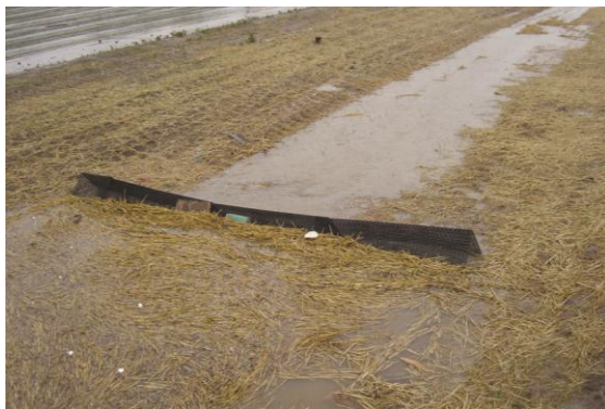
Excellent installation of a silt berm check dam.
