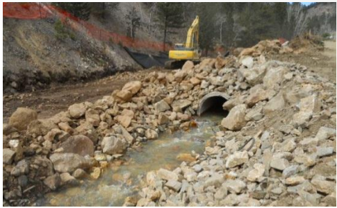
Good application of temporary culvert. Notice riprap approach to culvert
