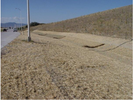
Excellent mulch application. Fibers should be crimped or disked into soil and should stand upright.
