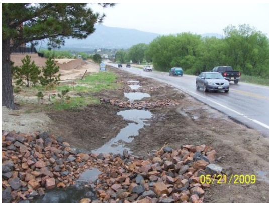
Excellent installation of rock check dams.
