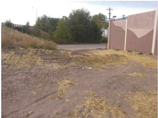
Poor mulch installation. Not enough mulch was applied and it was not anchored to the soil, which left bare areas.
