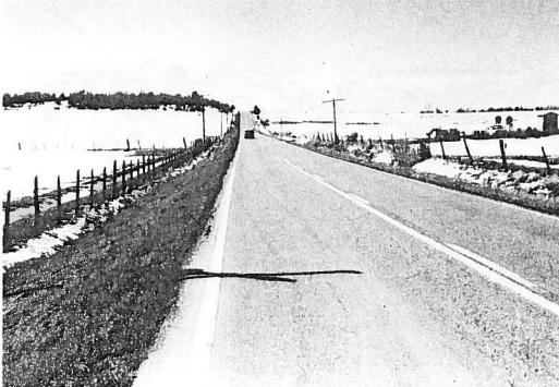
13. Looking west. Seasonal drainage is a problem along the right-of-way. Though not evident because these pictures were taken in late winter, water accumulate in ditches like the one on the left, causing maintenance time and expense to improve drainage. The proposed project will correct many of the problem by changing drainage slopes and cross culverts.
