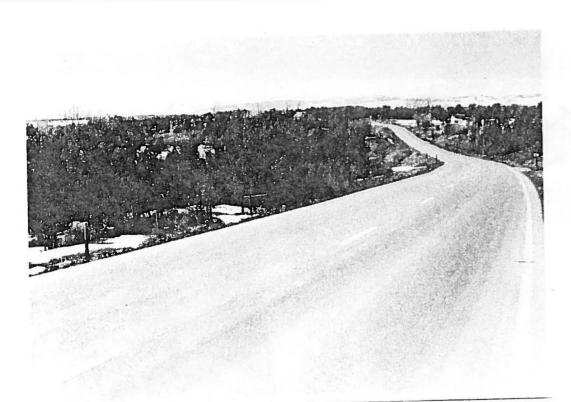
8. Looking northwest towards the La Plata Mountains. The problem which exists without adequate paved shoulder is evident when vehicles turn on and off the highway at the residential driveways. Vehicles which cannot pull off when slowing down cause others to pass where it is unsafe. At this particular spot you are coming over a hill when the driveway on the right occurs. The proposed project would construct 6-foot paved shoulders here.
