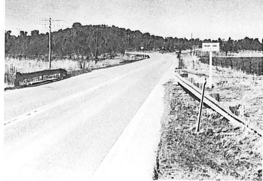
7. Looking south at the Morrison Canal ditch crossing. The narrow crossing is the cause of accidents involving the guardrail and vehicles which are limited to an unsafe section width here. Maintenance problems include guardrail replacement at the crossings and drifting snow caused by cross winds in the background of this photo.
