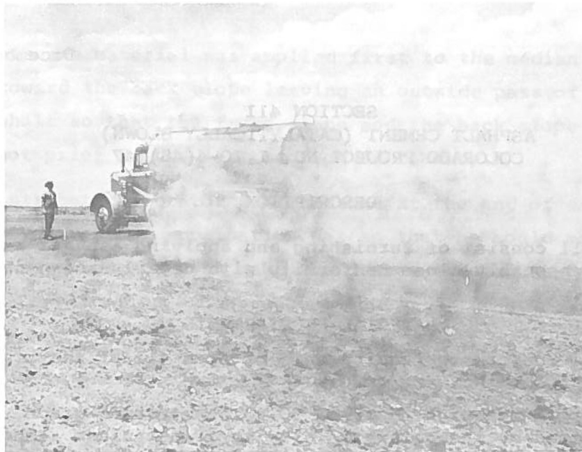
Figure 4. Distributor Applying Asphalt Membrane
