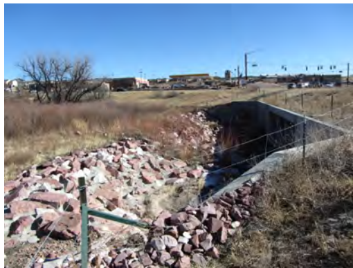
Photo #7: AZ -Jackson Creek (North Baptist Rd.)
