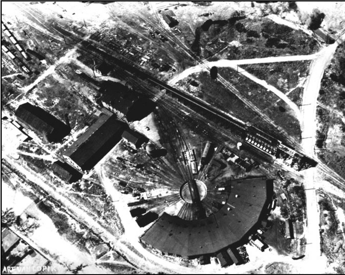
Figure 13. Aerial view of the Colorado Midland Roundhouse, circa 1939 (Pikes Peak Library District)
