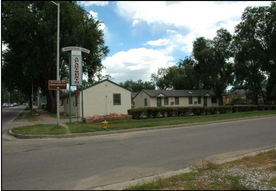
Figure 24. The Mountain Edge Apartments at 2032 West Cucharras Street, built in 1955. An early example of tourist-related facilities converted to multi-family, low-income residential dwellings
