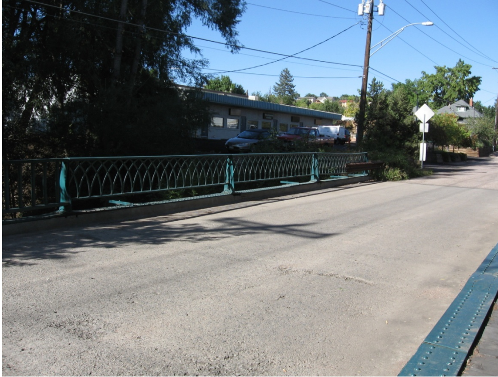
Figure 56. South 26th Street Bridge, 5EP3662
