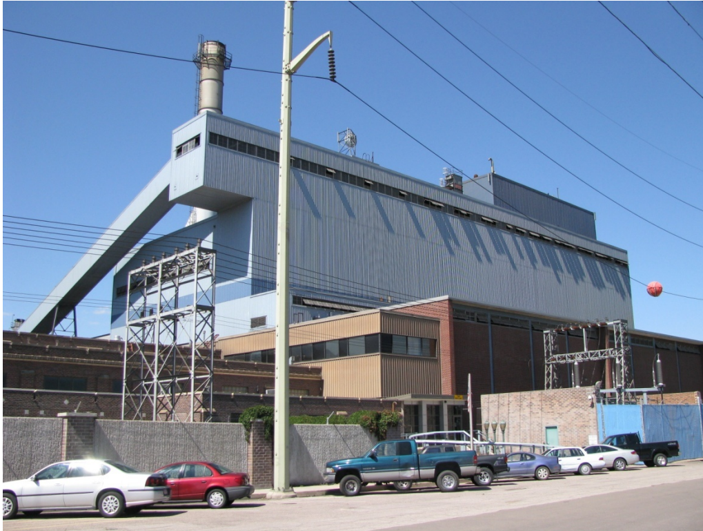
Figure 55. Martin Drake Power Plant, 5EP5360
