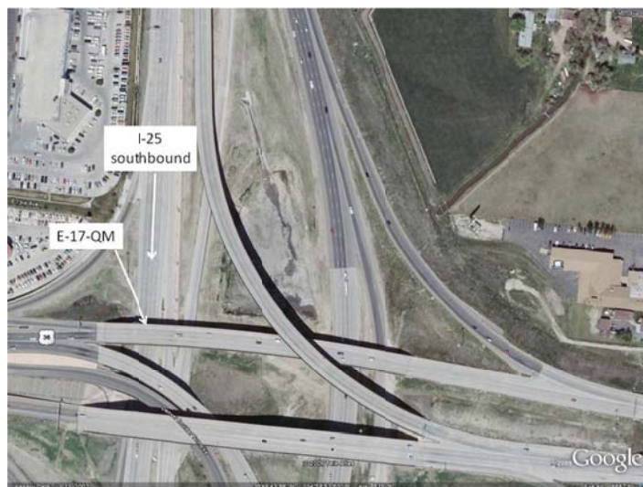
Fig 3.1 Bird's eye view on Bridge E-17-QM
