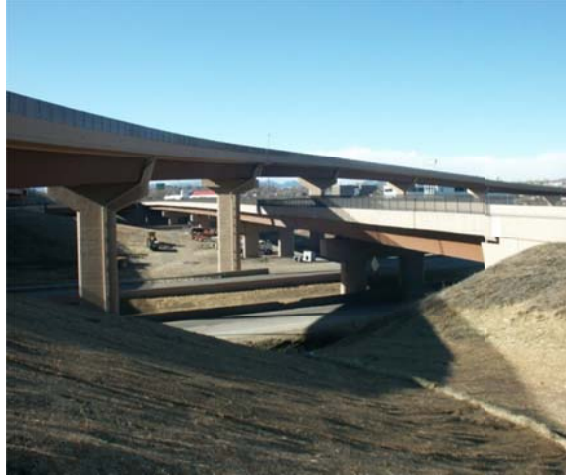
Fig 3.2 Side view of Bridge E-17-QM
