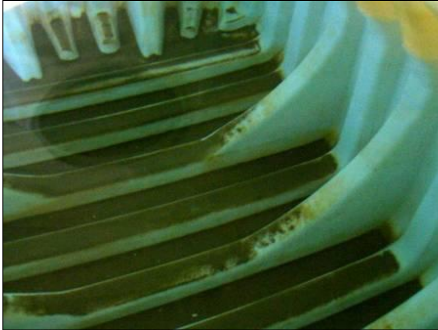
Figure 5. Green Sediment in the Lodge's Storage Tank Observed During the 2009 Sanitary Survey
