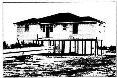
Figure 2.3. After Hurricane Hugo, many coastal homes in South Carolina were elevated by house movers, but almost none were relocated further from the water's edge. (Photo by R. Platt.)
