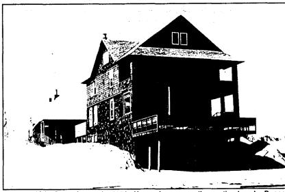
Figure 7.1(b). Same house in 1970. House is now partly on the beach. Dunes, boardwalk, and most neighboring houses along the oceanfront are gone. (Photo by R. Platt.)
