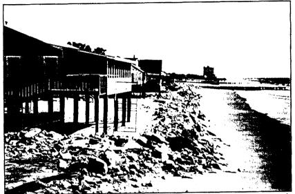
Figure 5.6. Six months after Hugo (March 1990), rebuilt homes stand at the water's edge behind makeshift private revetments. The structure in the foreground is elevated to NFIP standards, but no setback was imposed by state or federal authorities. The Holiday Inn stands on artificial fill in the distance. (Photo by R. Platt.)
