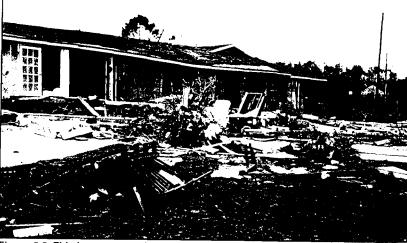
Figure 5.5. This house on the Isle of Palms was moved landward off its foundation by Hurricane Hugo. (Photo by R. Platt.)
