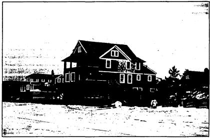
Figure 7.1 (c). By 1987, the dune line has receded behind the house, leaving it entirely on the beach. House was washed away on October 31, 1991. (Photo by R. Platt.)
