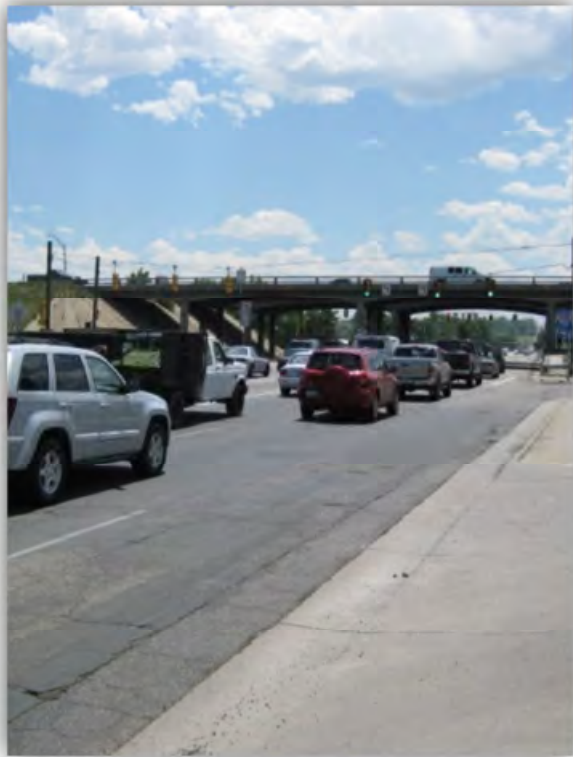
Kipling Street at eastbound I-70 ramps intersection
