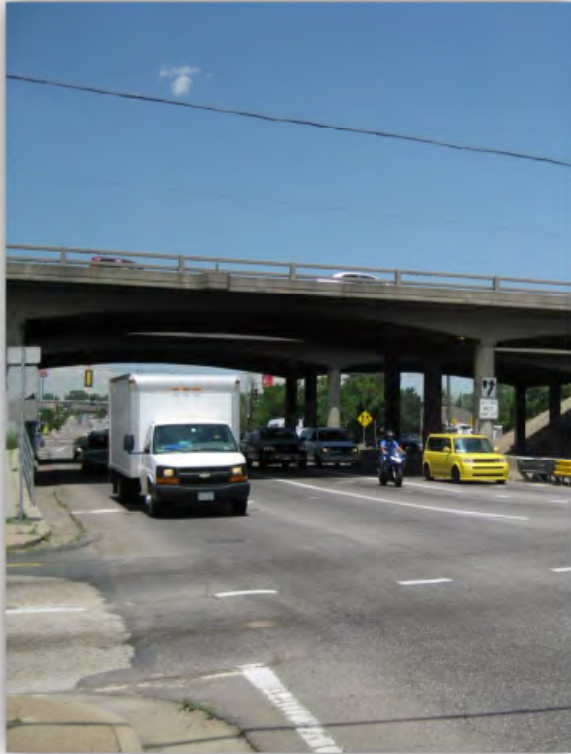
Looking north along Kipling Street towards I-70
