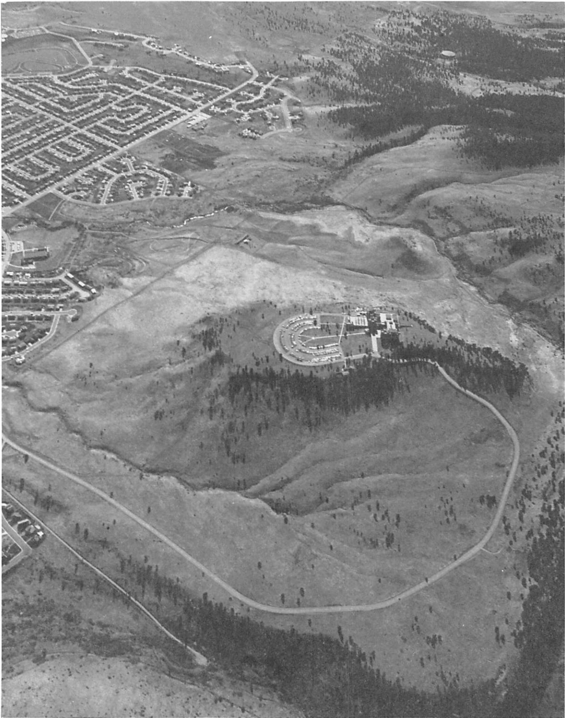
Figure 30. Slopes underlain by Pierre Shale such as those from NCAR, center, north to Chatauqua are vulnerable to landsliding when notched or "bench cut" for roadbeds or foundations (photo by NCAR).
