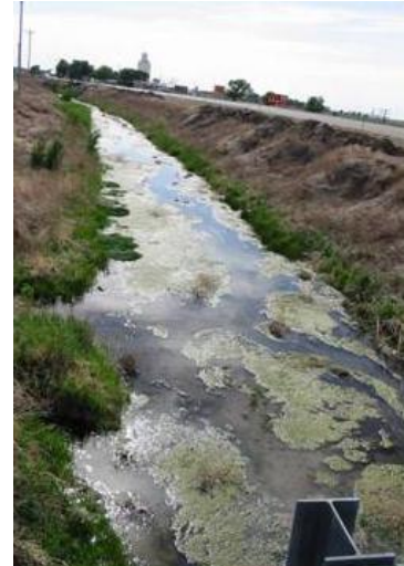
Irrigation Canal in the Study Area
