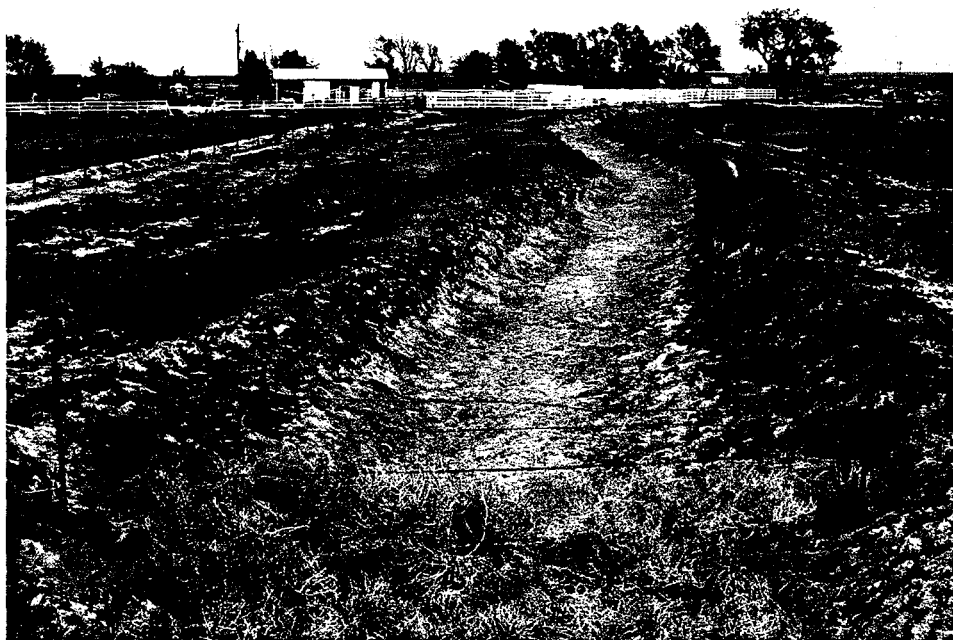
5PW192.1 Feature 1, canal. View east from county road.
