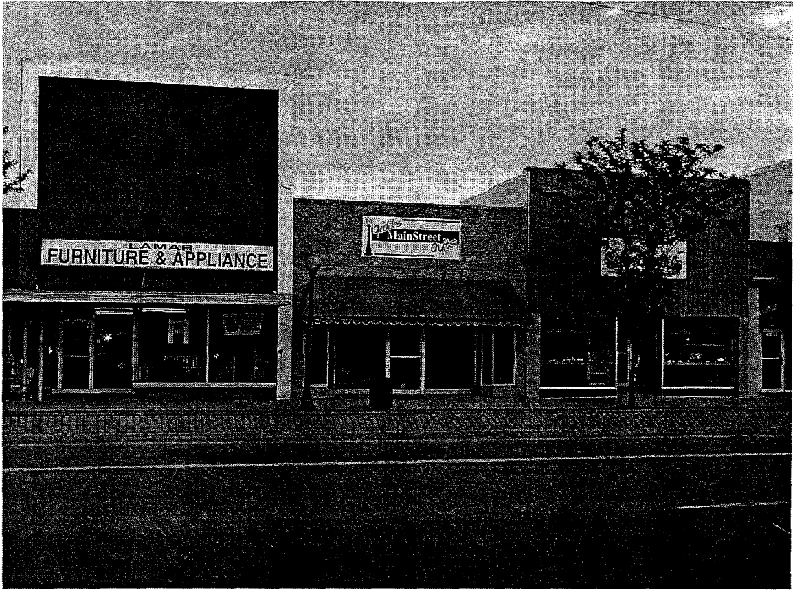
Figure 8: View east at the east side of Main Street between Beech Street (north) and Olive Street (south). Photo taken May 15, 2003. Note discontinuity in architecture and loss of historic integrity.
