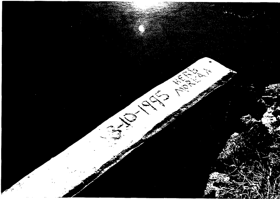
5PW191.2 "3-10-1995 Herb Morlan" scratched in upgraded concrete retaining wall.
