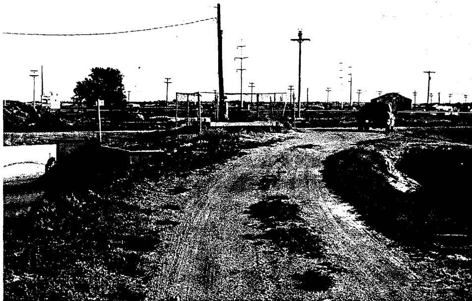
5PW191.2 Feature 2, presumed old ditch rider's road, view north. Most likely rebuilt after 1965 flood. Feature 1 to left.
