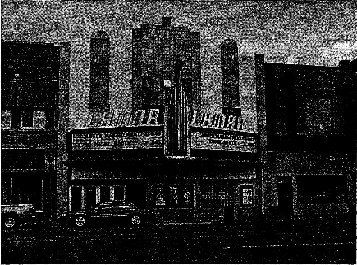
Figure 3: View east at Lamar Theater. Photo taken on May 15, 2003. Masonic Temple building is to right (south).
