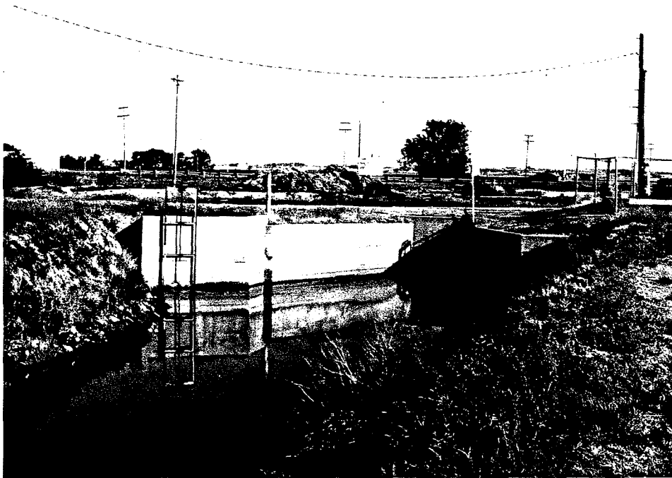
5PW191.2 Lamar Canal, view northwest of northern extent of Feature 1 and concrete retaining wall (c.1995).
