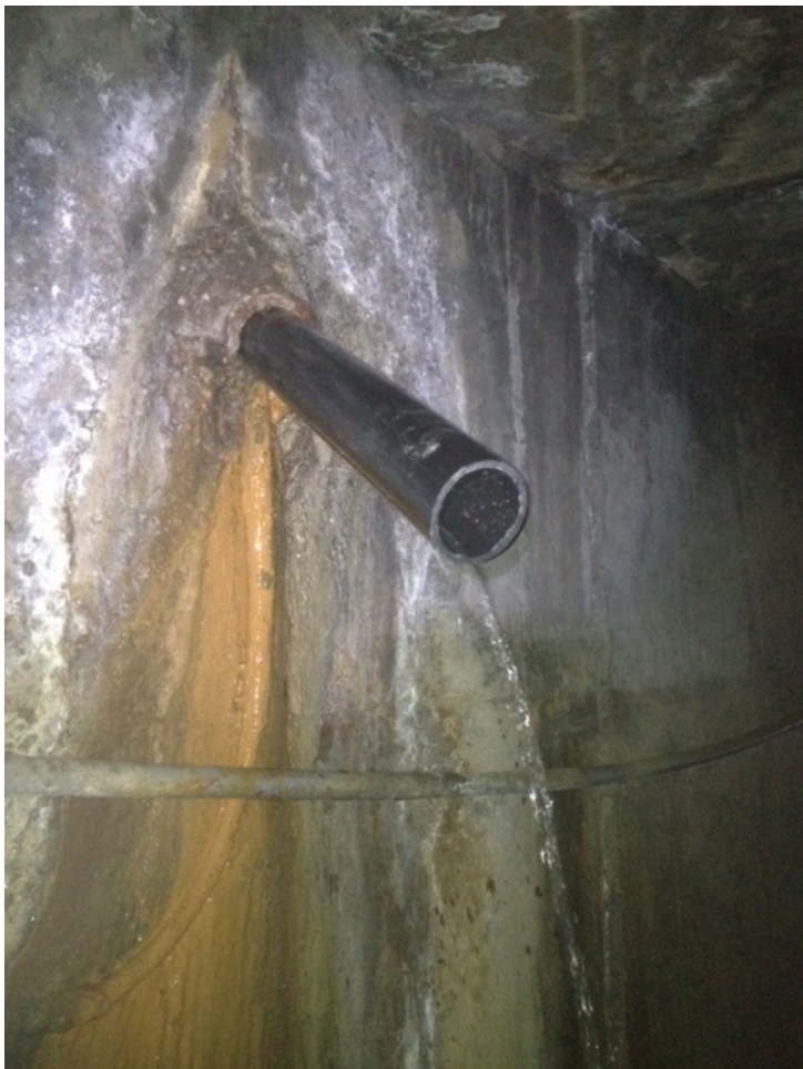
13. Northern Tunnel Discharge
