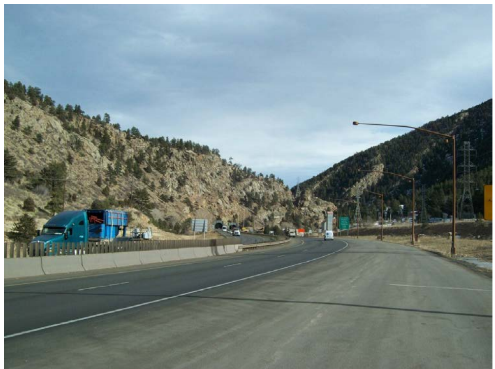
8. I-70 West of Twin Tunnels. Chain Station in Foreground
