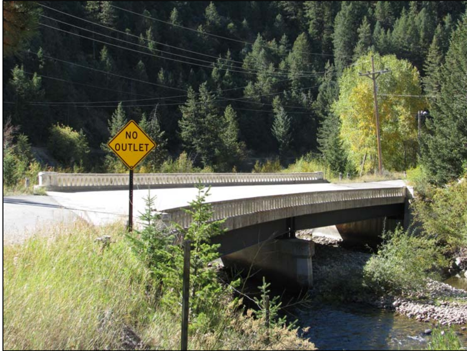
Figure 9. View southwest of U.S. 6/40 bridge, site 5CC1081, over Clear Creek.
