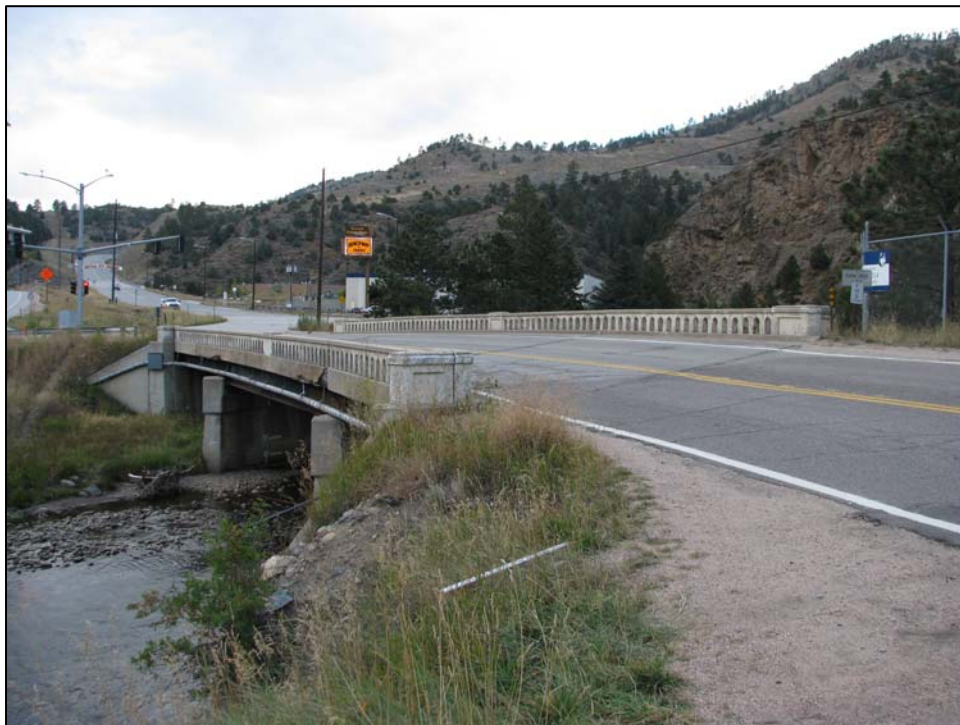
Figure 8. View northwest of 5CC1078, the U.S. 6/40 Clear Creek F-15-D bridge.
