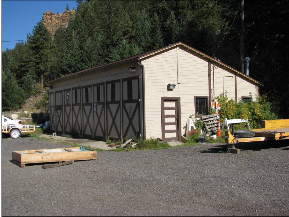
Figure 7. View of northwest and southwest elevations of the C&M Shop at the Idaho Springs Work Center (5CC698), facing east.
