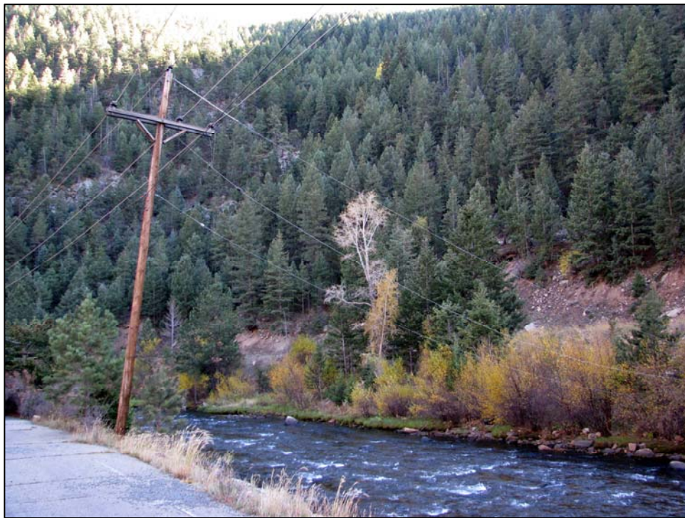
Figure 24. View southeast of the area once occupied by the Seaton Mountain Electric Company plant and flume (5CC1996). This photograph is an approximate replication of the view shown above in Figure 23.
