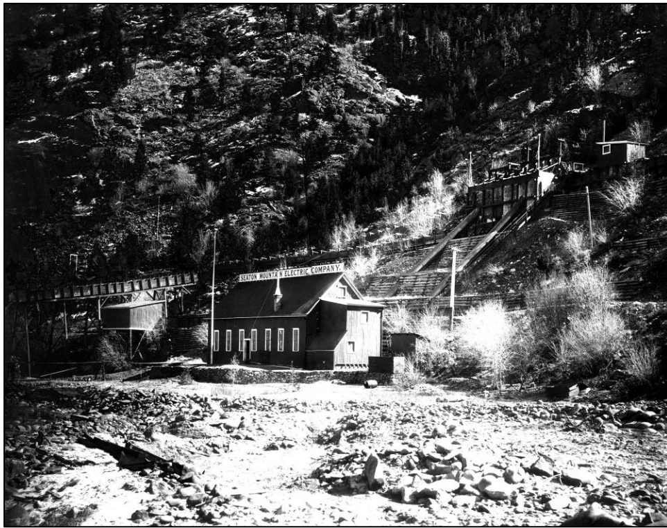
Figure 23. View southeast of the Seaton Mountain Electric Company plant and flume (5CC1996), circa early 1900s. (Photograph used by permission, Idaho Springs Heritage Museum and Visitors Center.)
