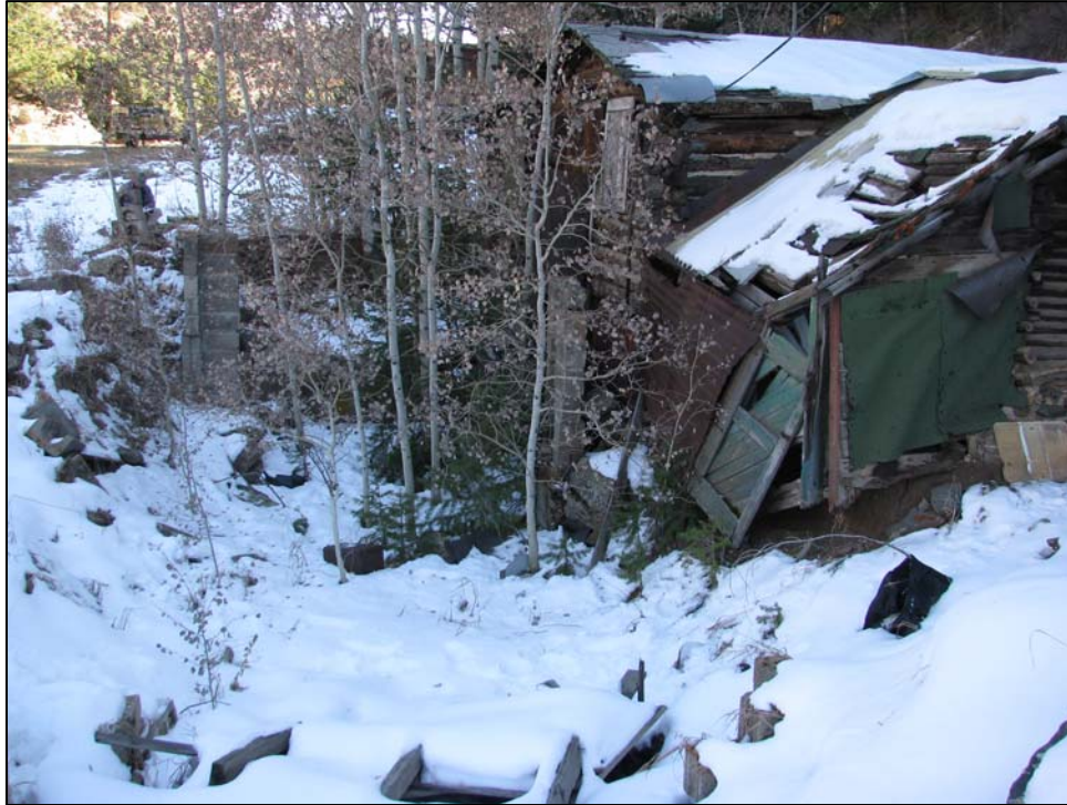
Figure 38. View east of the 1922 cabin at site 5CC2000.
