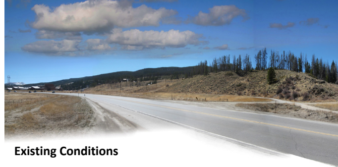
Figure 9 KOP 3 Looking South toward Breckenridge
