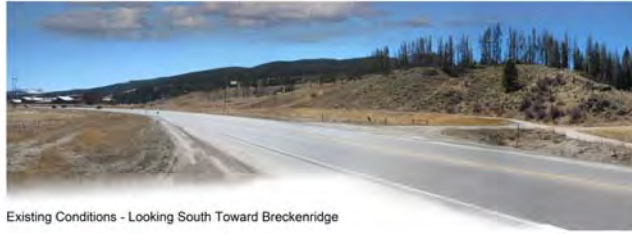
Existing Conditions - Looking South Toward Breckenridge
