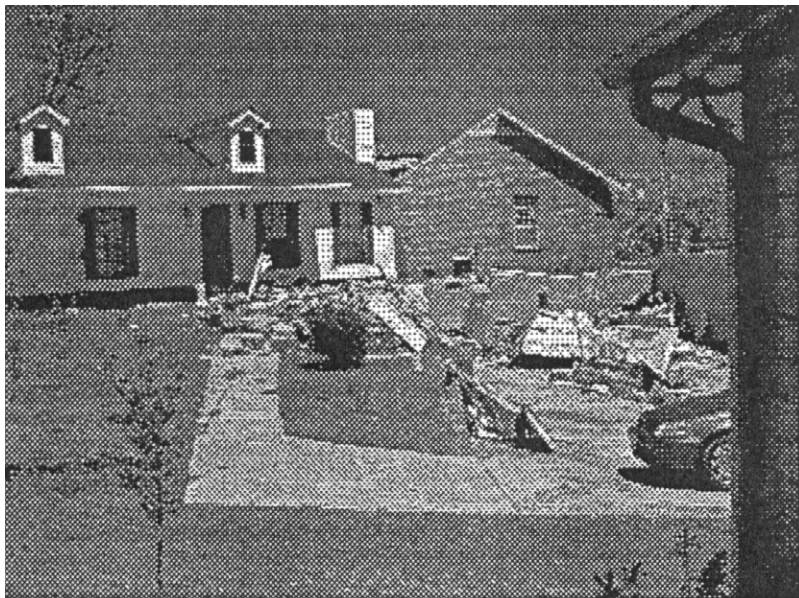
House pushed off foundation - Concord
