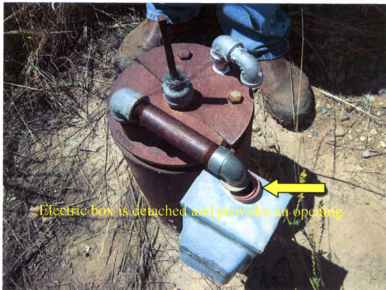
Attachment # 3 - Well 005: Conduit box is detached and provides an opening for potential contaminants.
