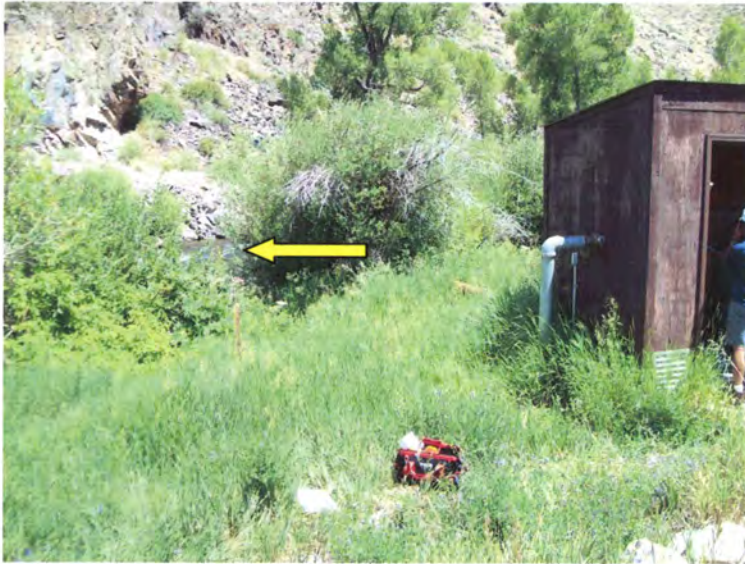
Attachment # 7 - Well 003: Approximately 25 feet from the Taylor River and has a static water depth of 36 feet
