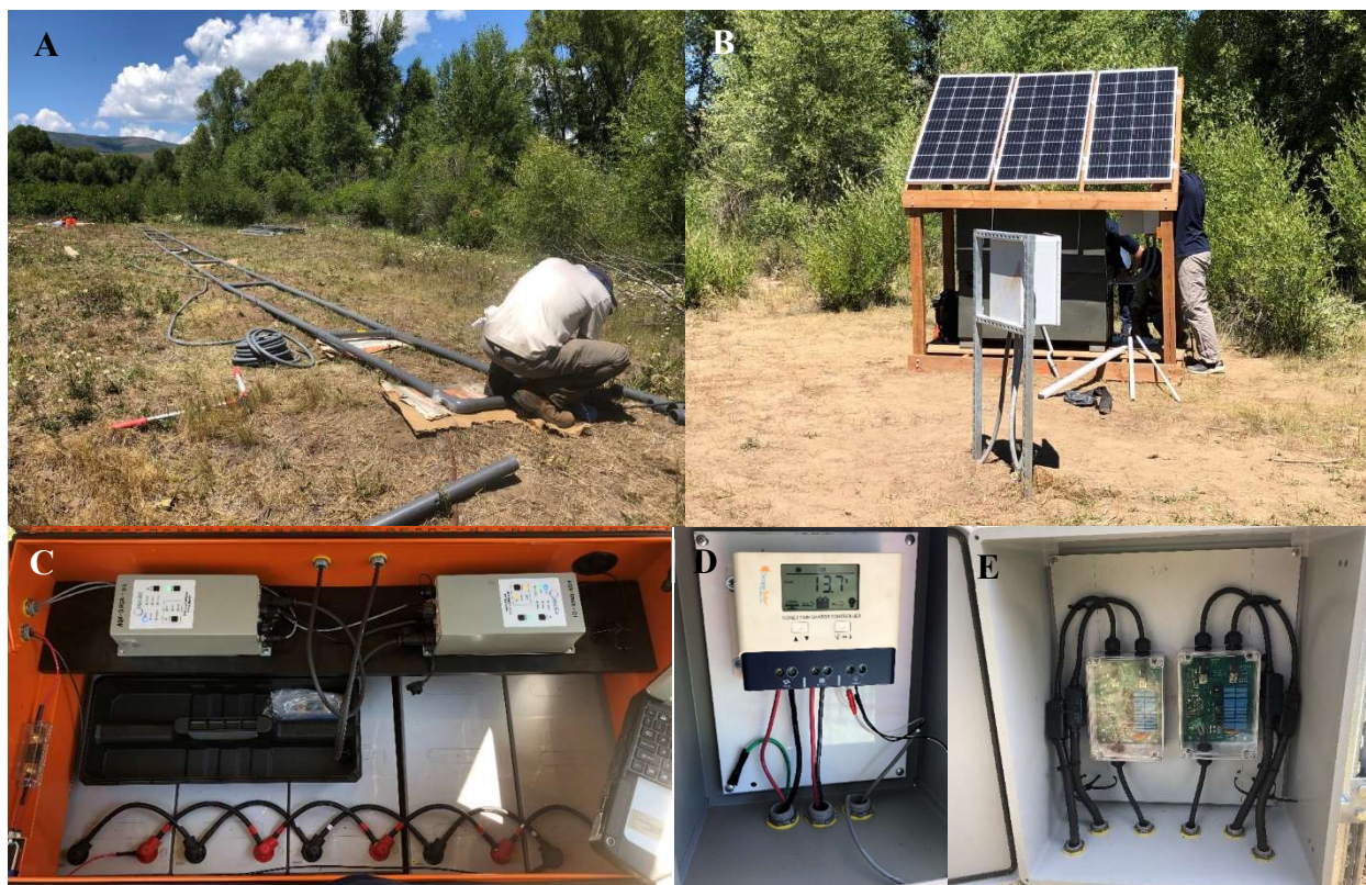
Figure 2.9. Antennas were constructed onshore prior to installation (A), as were the reader stations containing solar panels, (B) the battery bank powering the Oregon RFID ORSR readers (C), a charge controller (D), and a standalone housing unit for the antenna tuner boxes (B and E).
