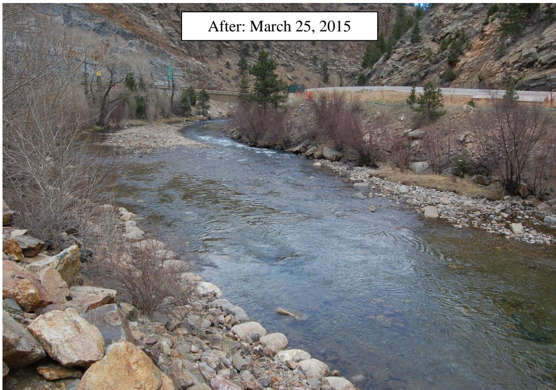
Figure 1.4. Post-construction photo of the downstream “low-intensity” stream site as part of the Twin Tunnels project on Clear Creek.
