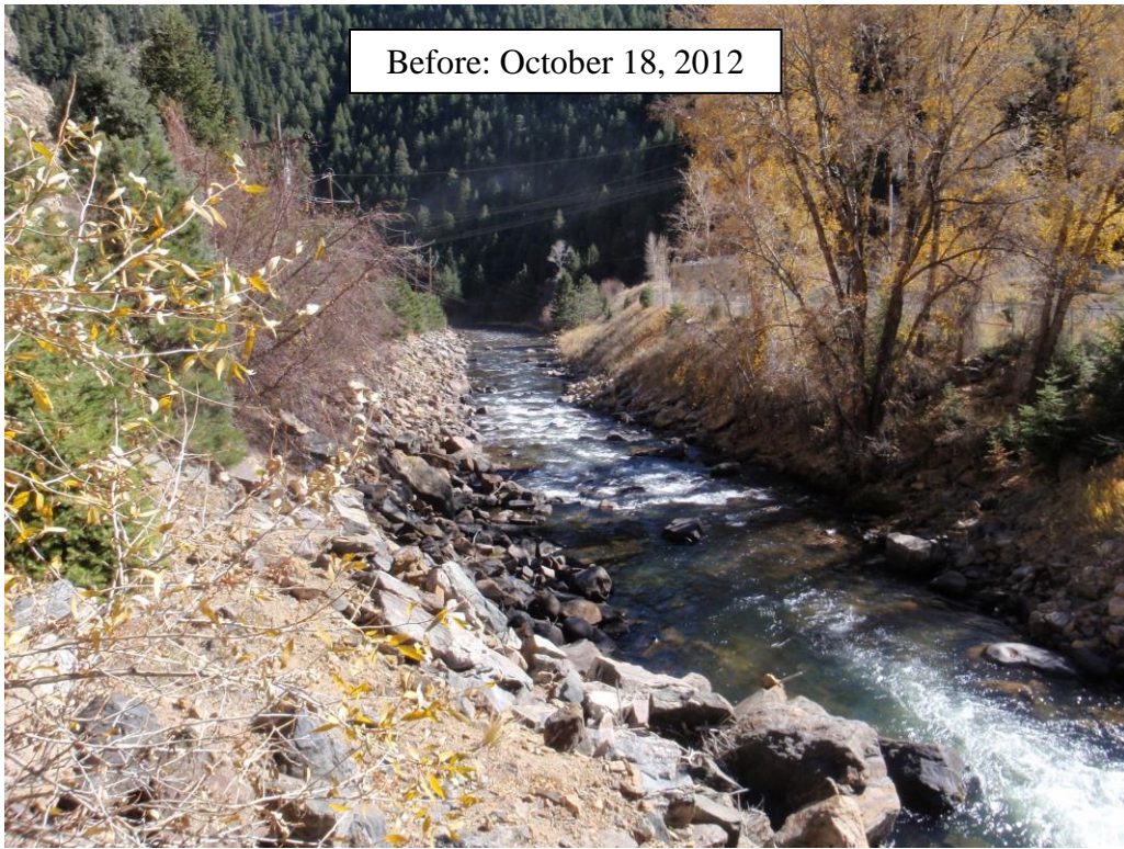
Figure 1.1. Pre-construction photo of the highly-confined “high-intensity” stream site as part of the Twin Tunnels project on Clear Creek.
