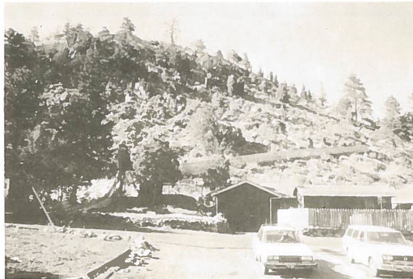
Below: A response to the above problem - this concrete wall diverts acidic runoff produced by the tailings on the top of the hill away from homes.
