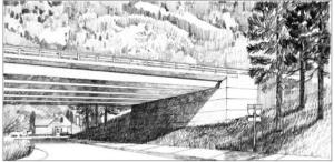
$C \mid A$  retrofit design for the facility shown above would remove slope paving and incorporate guidance for the design of bridge structures, planting, and pedestrian connections.
