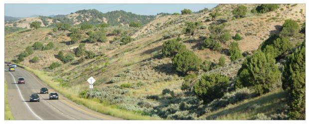
D / Utilizing variable slopes through the length of an embankment mimics the natural patterns found in the
