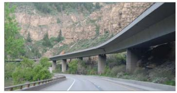
C / Elevated roadways will minimize disturbance on steep slopes.
