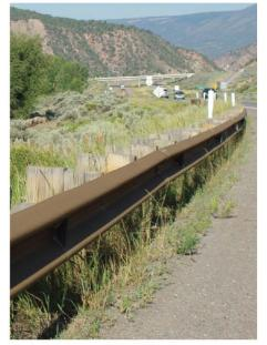
A / Self-weathering Type 3 Guardrail W Beam should be used for guardrails throughout this segment.
