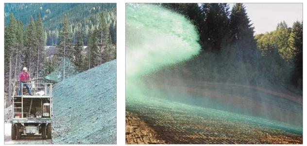
A | Mulching should be used to reduce dust and erosion impacts and promote successful revegetation.
