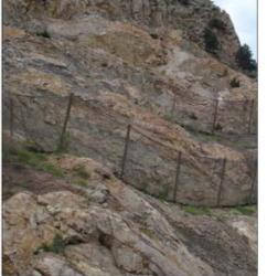
D | Rock fall protection devices, when required, follow existing contours, and reduce visual clutter.
