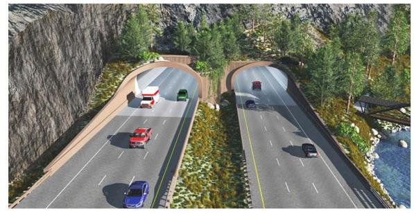
*C*/ *The transportation facility at the Twin Tunnels aids in rock fall protection by incorporating rock fall protection into the design of retaining wall, noise wall, grading and landscape.*
