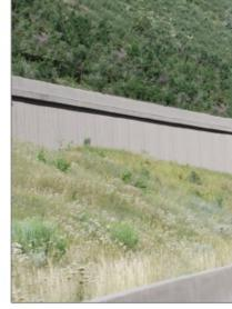
*C* | Incorporate earthwork solutions in conjunction with structured retaining to limit the height of retaining walls.
