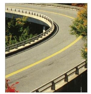
*C* / Utilizing attached metal rails on bridges rather than concrete barriers adds to the transparency and thin appearance of the span.
