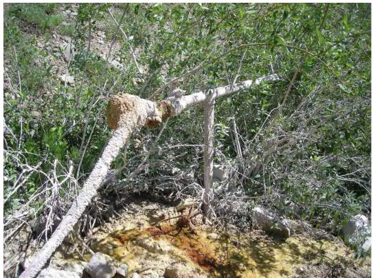
**Figure 20.** Close up photograph of Rico Drill Hole Group pipe, note junction of horizontal pipe with sloping hose. The precipitate on the ground is formed from leaking water at the pipe-hose junction.
