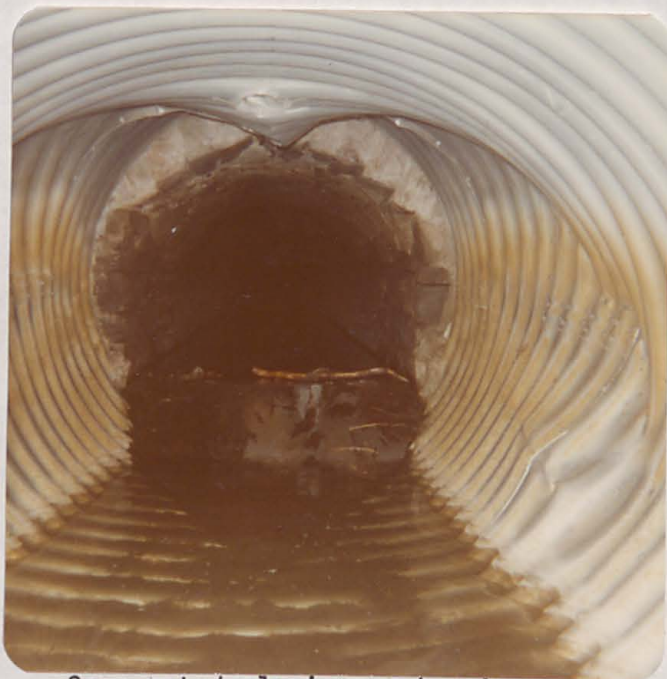
Corrugated aluminum extension 5' diameter, 60' long, added to masonry conduit in 1978
