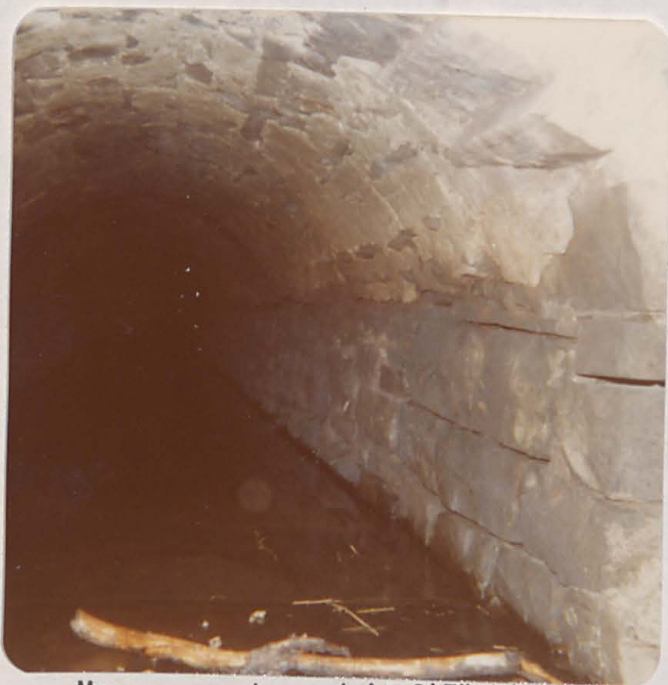
Masonry arch conduit 3'7" high, 5' wide, 140' long
