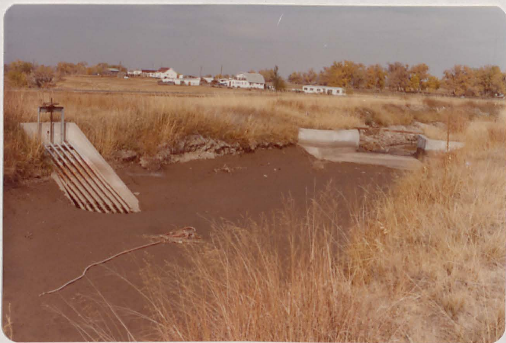
Parshall flume just downstream from Lonetree Dam measures flow in Home Supply Canal going past Lonetree Reservoir. Wasteway in front of flume can divert water to Lake Ditch Canal.
