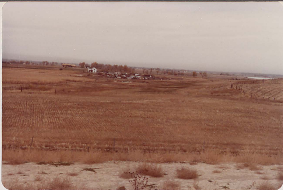
View from left side of spillway crest. Note house in flood plain and Ryan Gulch Lake in background.
