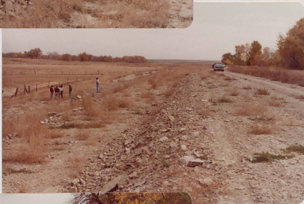
Tile drains under embankment have stabilized this old marshy area
