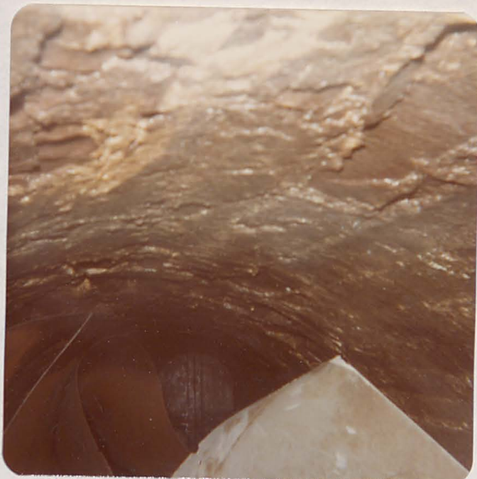
Metal fins below slide gates for improving flow characteristics
