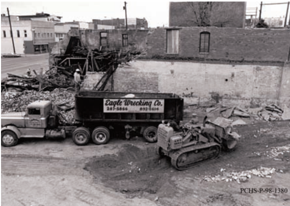
Figure 1.13. Excavation work was one of the first tasks in the construction of the Sangre de Cristo Arts Center, a long-anticipated addition to downtown Pueblo. (photo courtesy of Pueblo County Historical Society, PCHS-P-98-1380, John Suhay Collection)
