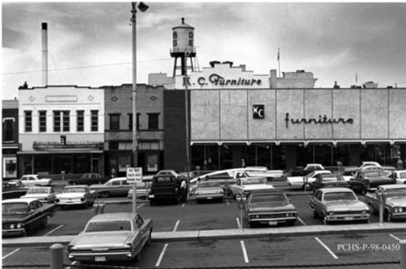
Figure 1.11. In an effort to compete with suburban strip malls, the City Council approved downtown parking lots. This one, at the 300 block of Santa Fe Avenue, offered parking but not the same convenience and proximity to stores as shoppers enjoyed at Midtown, Belmont, or Sunset Park shopping centers. (photo courtesy of Pueblo County Historical Society, PCHS-P-98-0450, John Suhay Collection)
