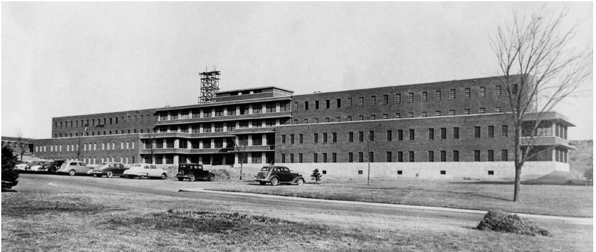
Figure 2.3. This image of the Female Building at the Colorado State Hospital was taken December 26, 1950. The four-story, brick, modest International Style building features a central bay with strong horizontal elements and recessed windows. (photo courtesy of Pueblo City-County Library District, Western History Collection)
